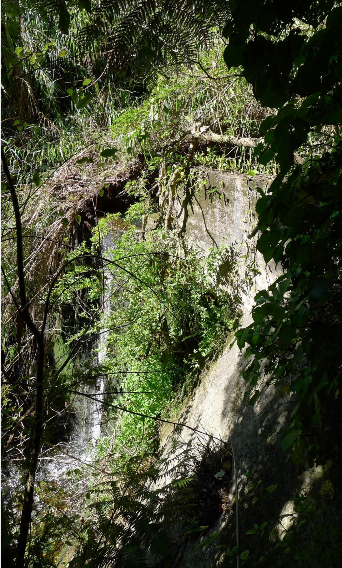
Figure 39. View towards downstream face of dam across eastern buttress
