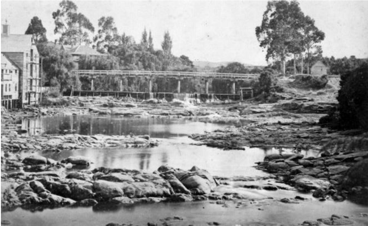
Figure 19. A braced timber dam/weir across the Mahurangi River. Water from the dam drove the flour mill to the left via a flume and waterwheel. In 1905 the Wilsons cement company concrete weir replaced this structure. Source unknown.
