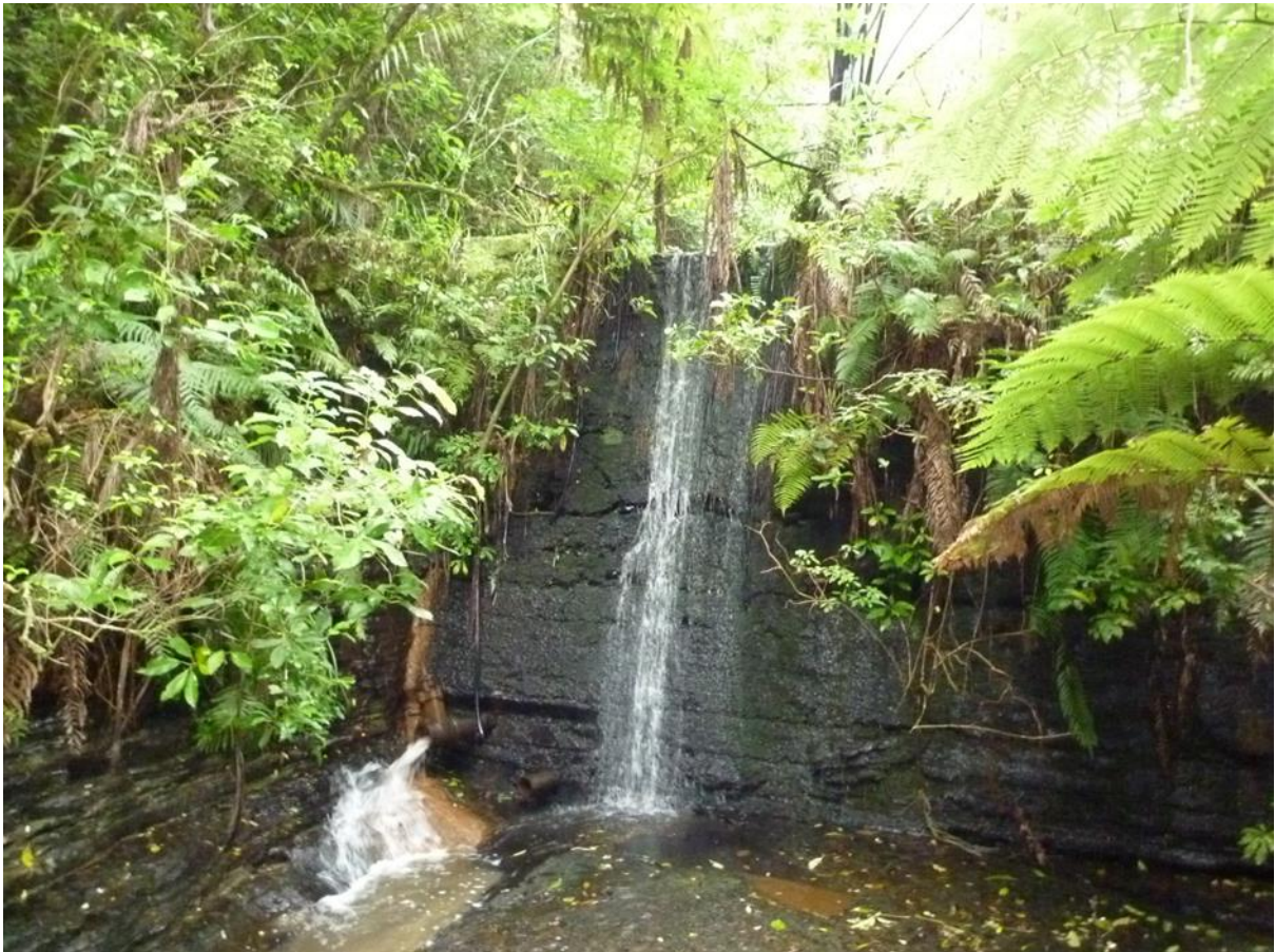
Figure 14. Dam 5 on the Mangakura Stream. WCS.
