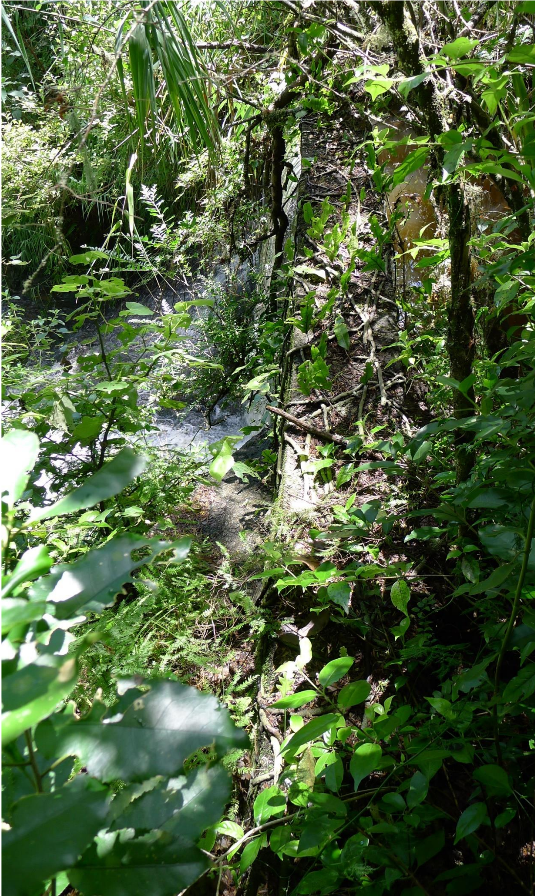
Figure 38. Top of dam from eastern abutment
