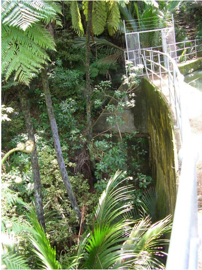
Figure 16. Right abutment of dam 3, showing buttress. WCS
