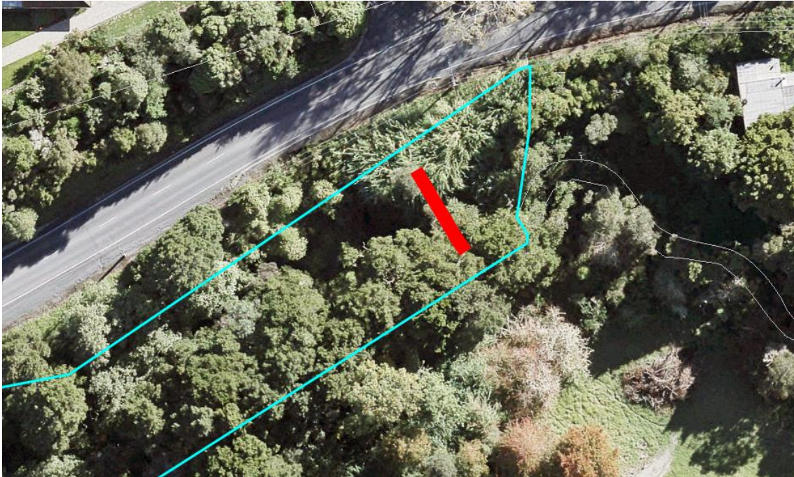
Figure 7. Approximate location of the dam and boundaries of the esplanade reserve adjacent to Sandspit Road. Auckland Council Geomaps image.
