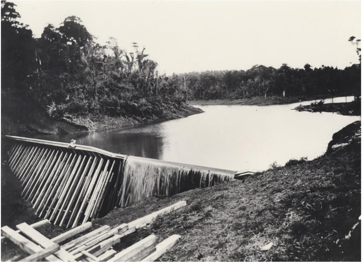
Figure 24. The timber auxiliary dam upstream from the Waitakere dam. Source: Walsh Memorial Library, The Museum of Transport and Technology (MOTAT) 06-655 (see also Offer p40).
