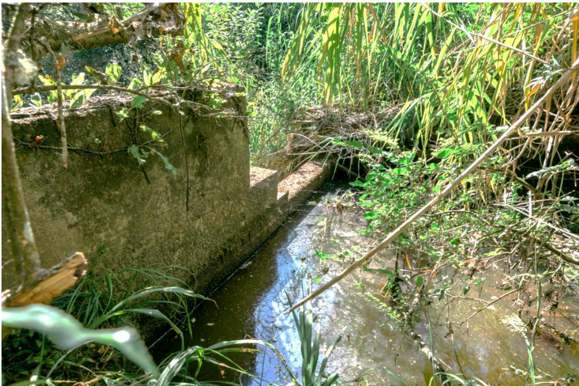
Figure 34. Downstream face of dam with water flowing over spillway into stream below.
