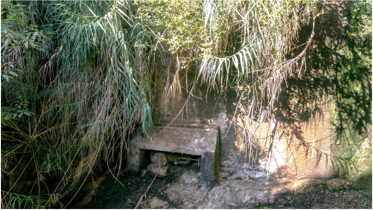
Figure 36. Front/downstream face of dam showing outlet valve and housing. Photograph: Jay Farnsworth (drone photo).
