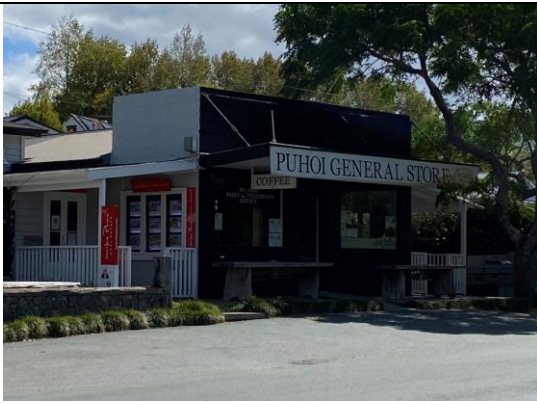
Pūhoi store, site visit, 2022
