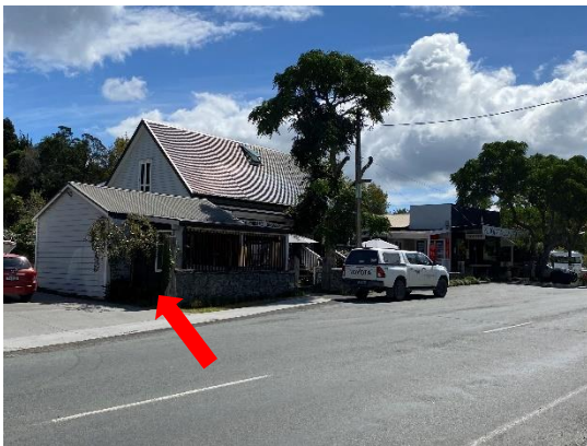
Wharf shed, site visit, 2022
