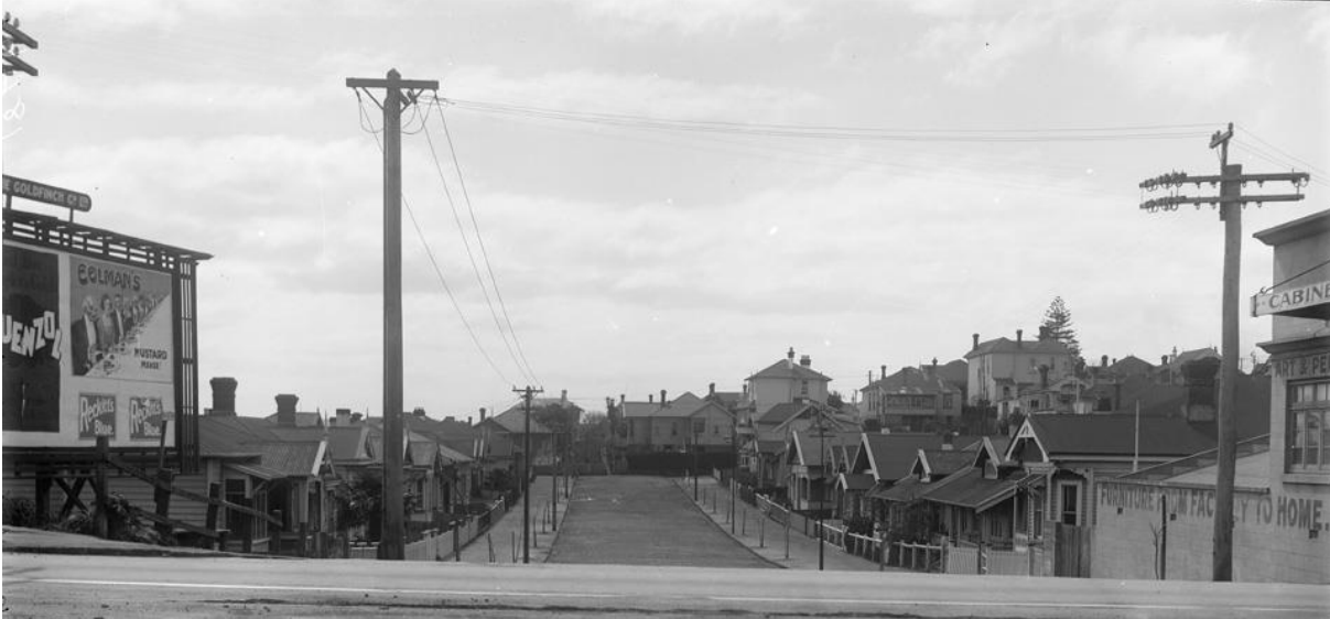
Figure 3: Parkfield Terrace from Khyber Pass, 1929 (Auckland Libraries Heritage Collections 4-1846)
