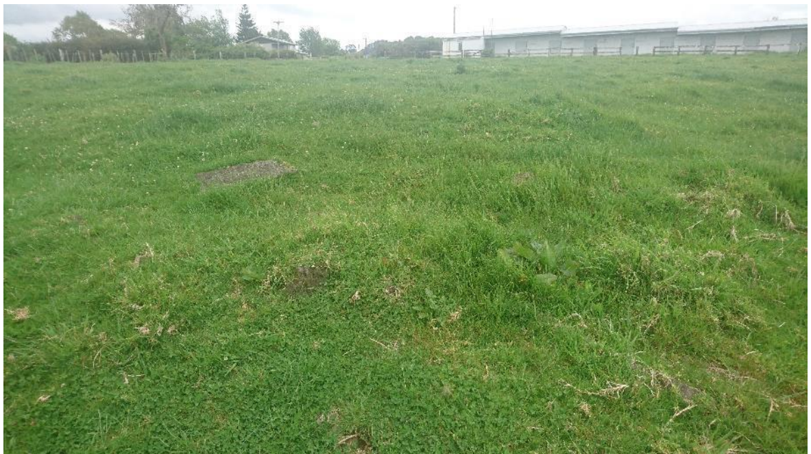
PLATE 8: PARTIALLY BURIED RUBBLE FROM PREVIOUSLY REMOVED BUILDING WEST OF HOUSE
