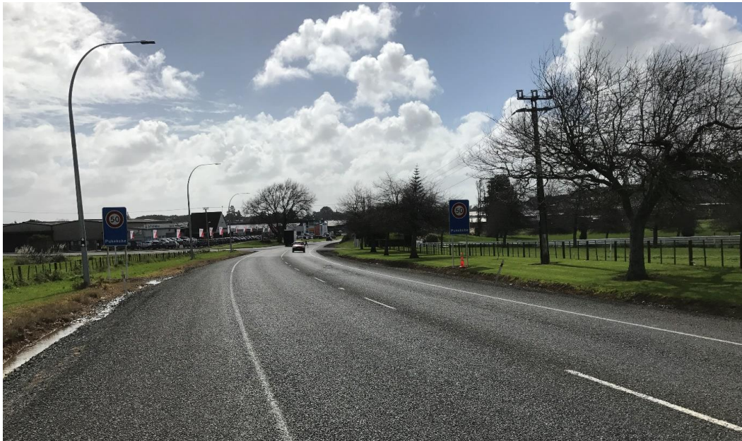
Photograph 1: Northern direction along Buckland Road (northern end)
