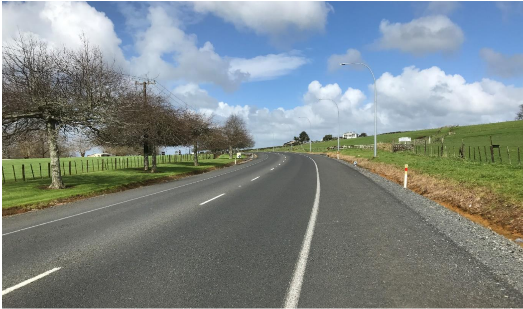
Photograph 2: Southern direction along Buckland Road (northern end)
