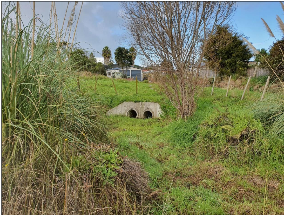
FIGURE 7: Dry detention pond outlet.
