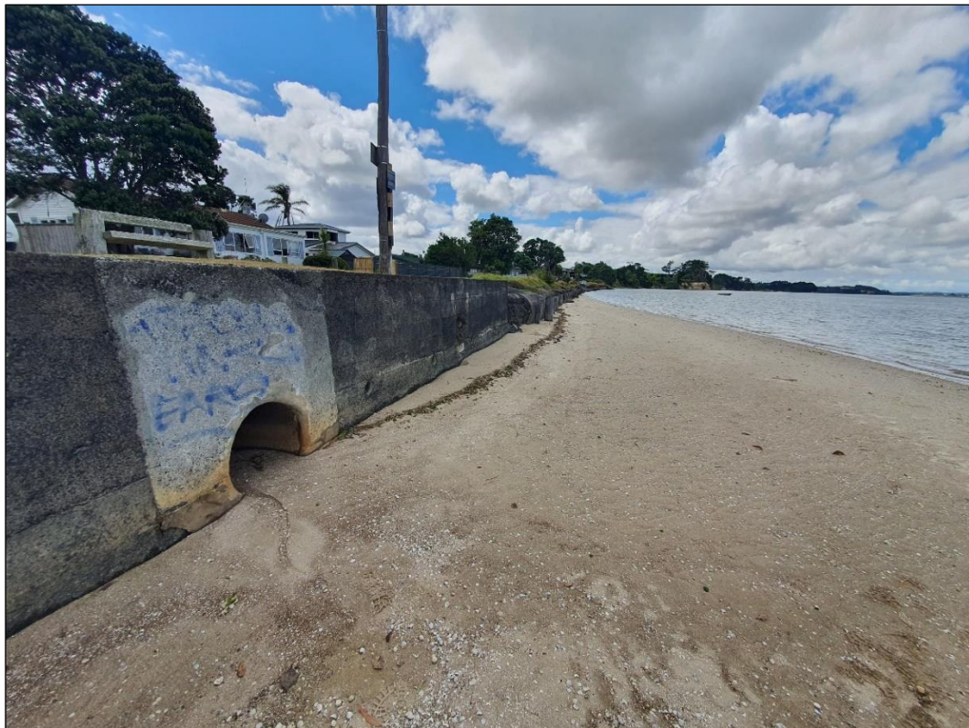
FIGURE 10: Stormwater outfall at Glenbrook beach.
