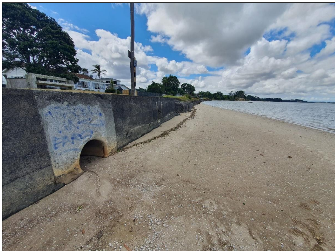
FIGURE 10: Stormwater outfall at Glenbrook beach.
