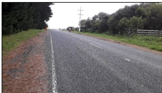
Eastern Site Frontage, facing North
