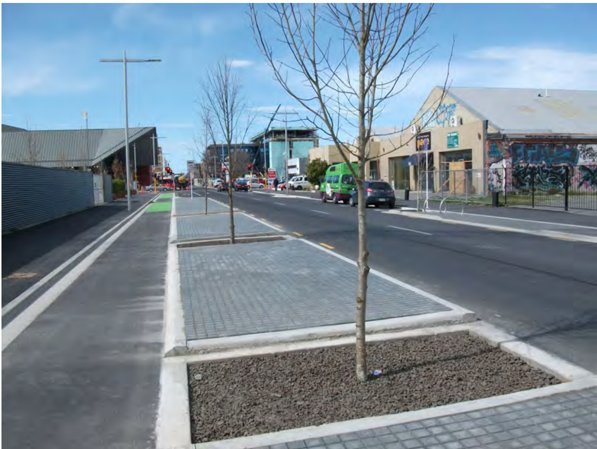
Figure 4-5: One-way separated cycleway – horizontal separation – Tuam Street, Christchurch (photo: Jeanette Ward, via NZTA website)
