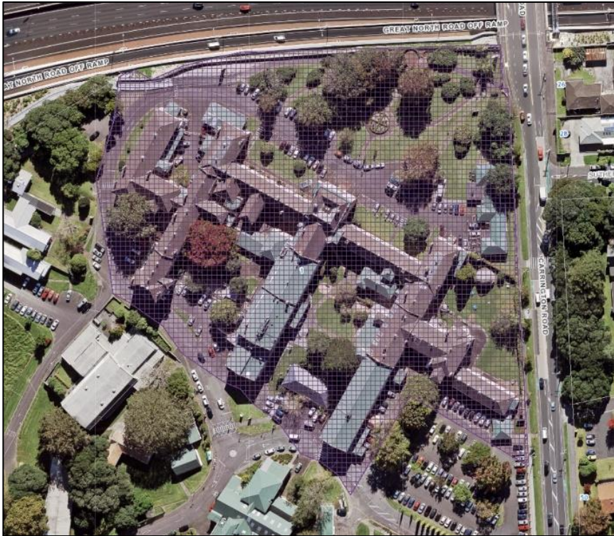
Former Oakley Hospital Main Building and Extent of Place in the Auckland Unitary Plan
