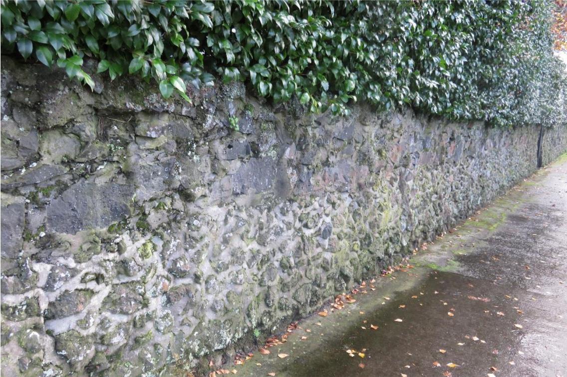
Figure 27: 153 Gillies Ave boundary wall along Brightside Road (south elevation). Note the two distinct layers to this wall, with smaller rubble stones in the lower half and larger cut stones in the upper half – indicating a later height increase.
