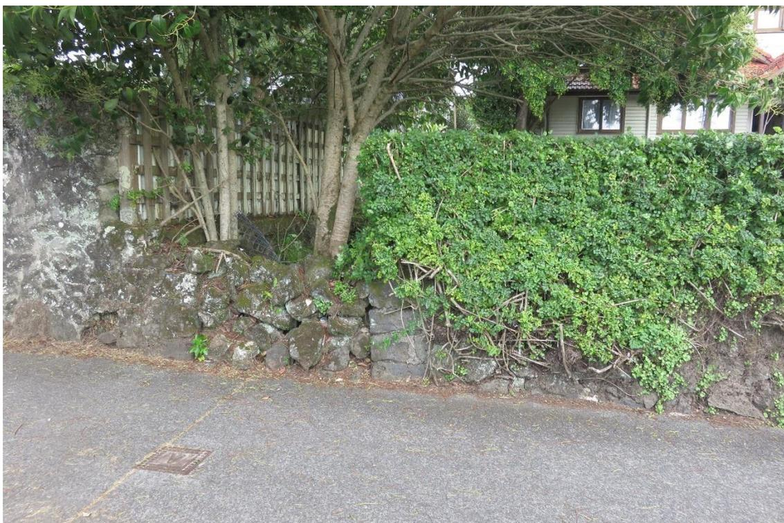
Figure 20: The wall is partially collapsed at the south-eastern corner of 149 Gillies Ave.
