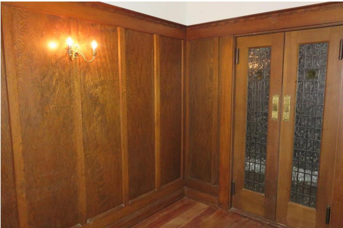
Figure 84: The entrance vestibule retains its clear-finished timber panelling.
