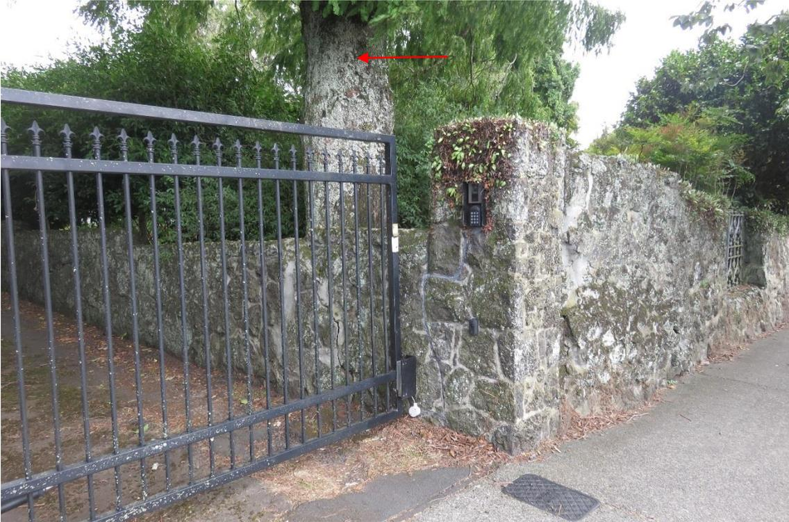
Figure 23: Historical stone pier and modern steel gate to the driveway of 151 Gillies Ave. The stone wall continues into the property along the driveway – note the severe cracking in the wall and heaving in the asphalt caused by the large dawn redwood tree (indicated) behind.
