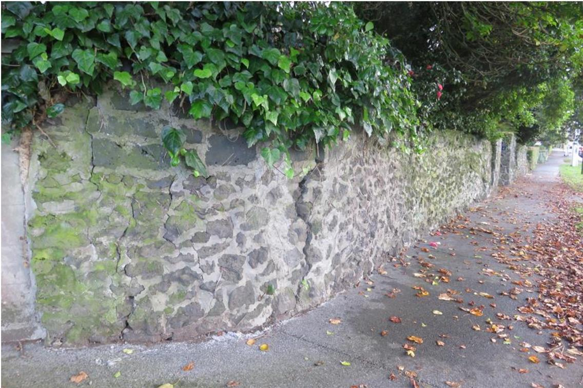
Figure 25: Severe cracking at the south-eastern corner, likely due to the large puriri and ivy behind.
