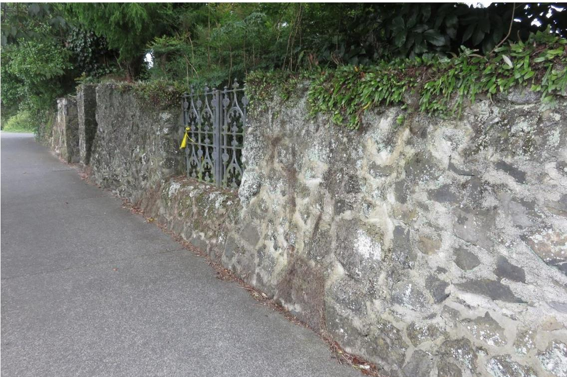
Figure 22: Step-down in wall with decorative metal railing. Note vegetation growing over the top of the wall.
