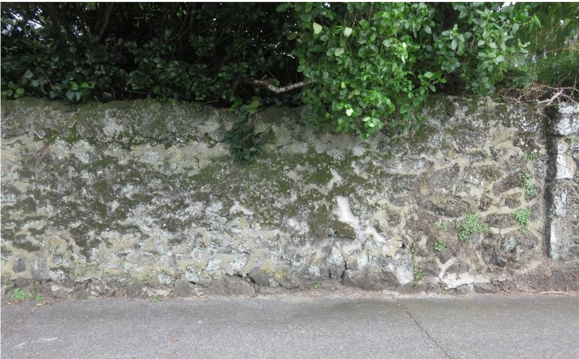
Figure 24: Stone wall to 153 Gillies Ave. This wall has settled, heaved and been variously repaired over time, resulting in a very undulating surface.
