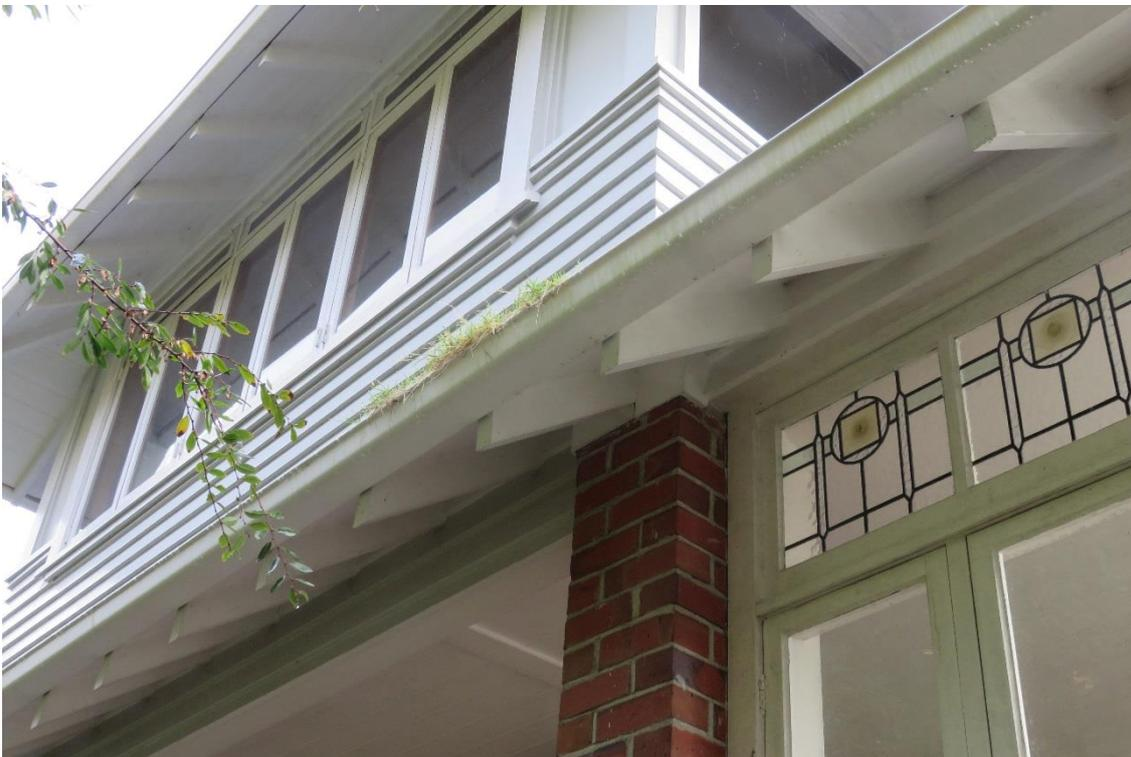
Figure 52: Detailing of the house's front façade. The building is generally in good condition although the gutters need frequent cleaning.
