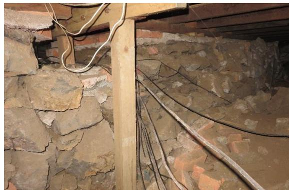
Figure 36: The original building retains its very substantial basalt foundational perimeter wall and subfloor support.
