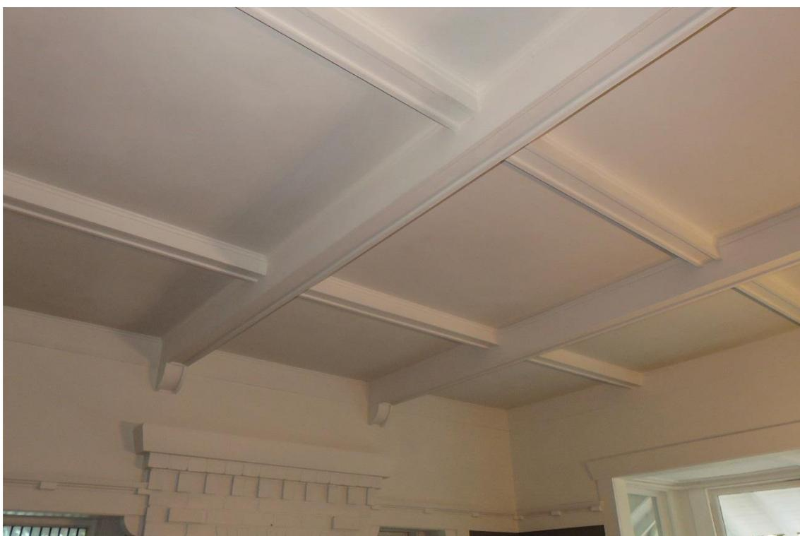
Figure 86: Timber-panelled ceilings are typical of the style and period.
