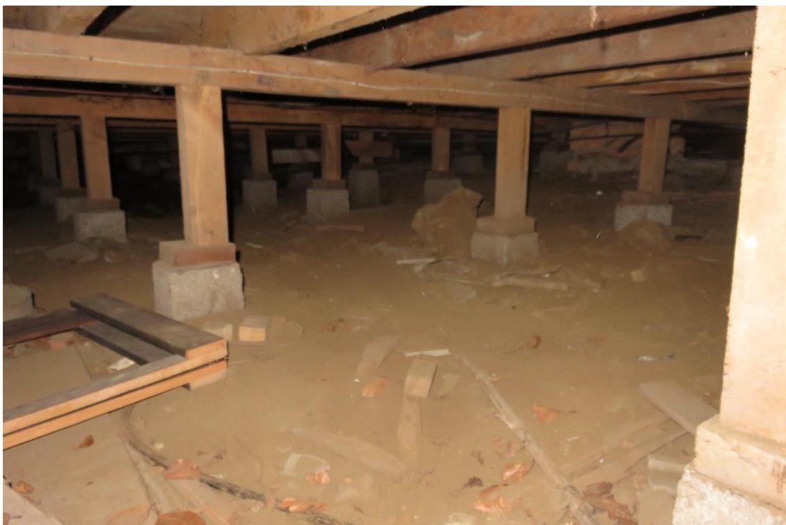
Figure 82: The substructure of the house appears in good condition.
