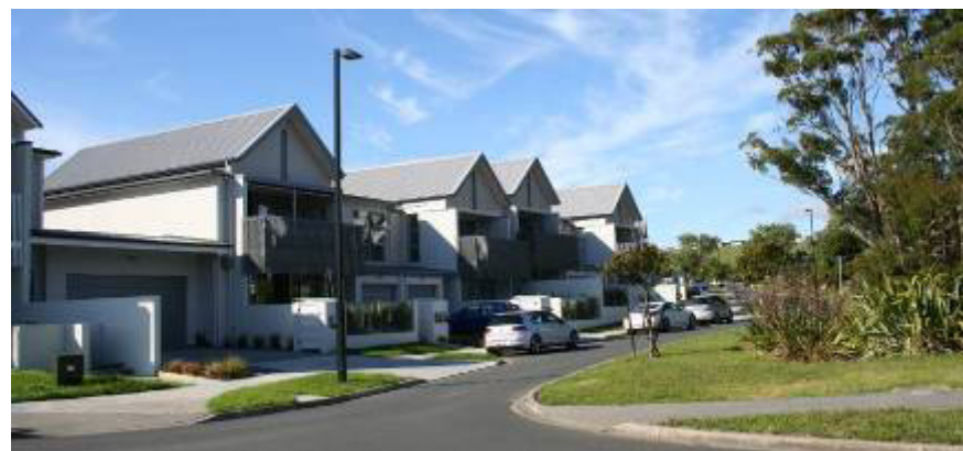
Photograph 23: Another Millwater example of compact housing, demonstrating skilful stepping of structures up the inclined landform,
