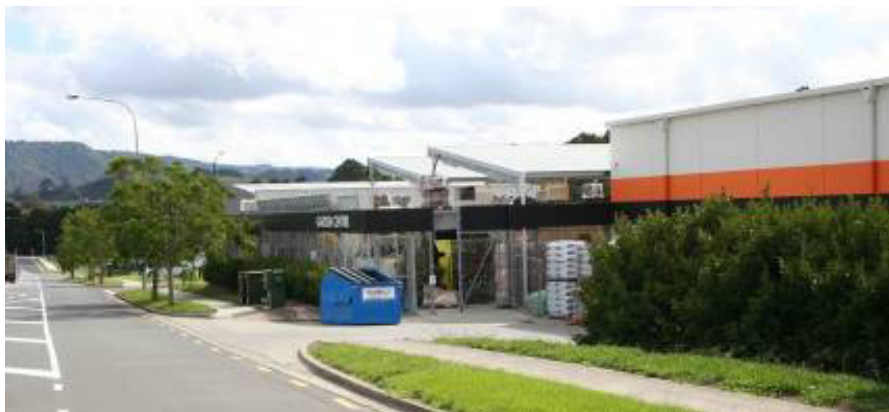
Photograph 7: The recently developed Mitre 10 store on Mansel Drive. Roadside vegetative screening and verge street trees are relatively effective in buffering the presence of this loading area.
