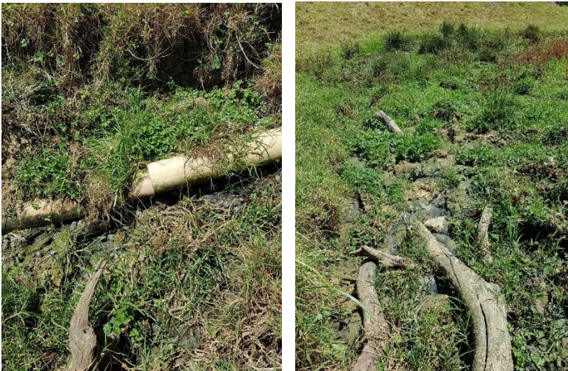
Plate 5.3. Watercourse 2 (southern watercourse). Images showing the broken pipe in the upper reaches (left) and water pooling in pug marks downstream (right).
