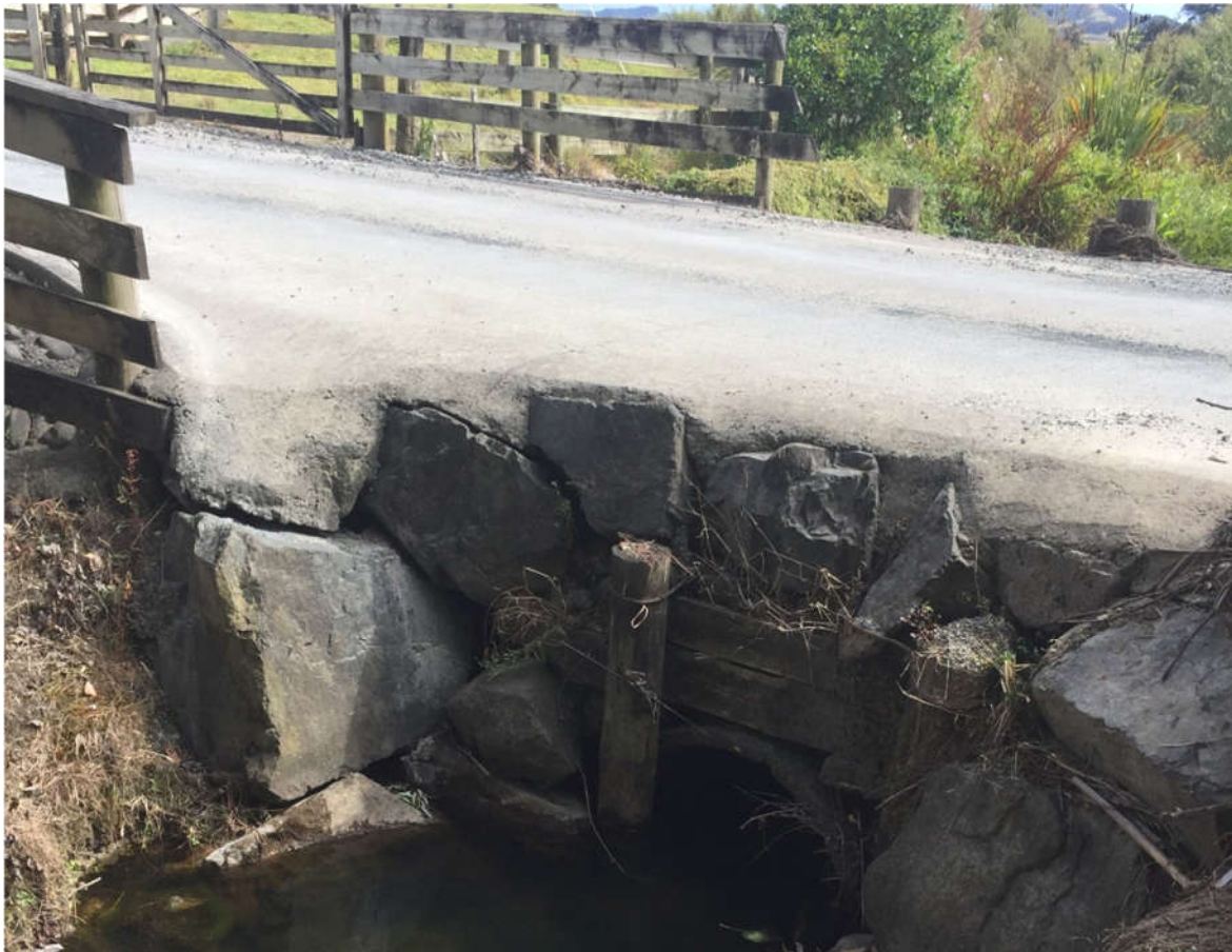
Figure 15 – Culvert at the end of Sanderson Road (Taken by J Curtis 14.01.2017)
