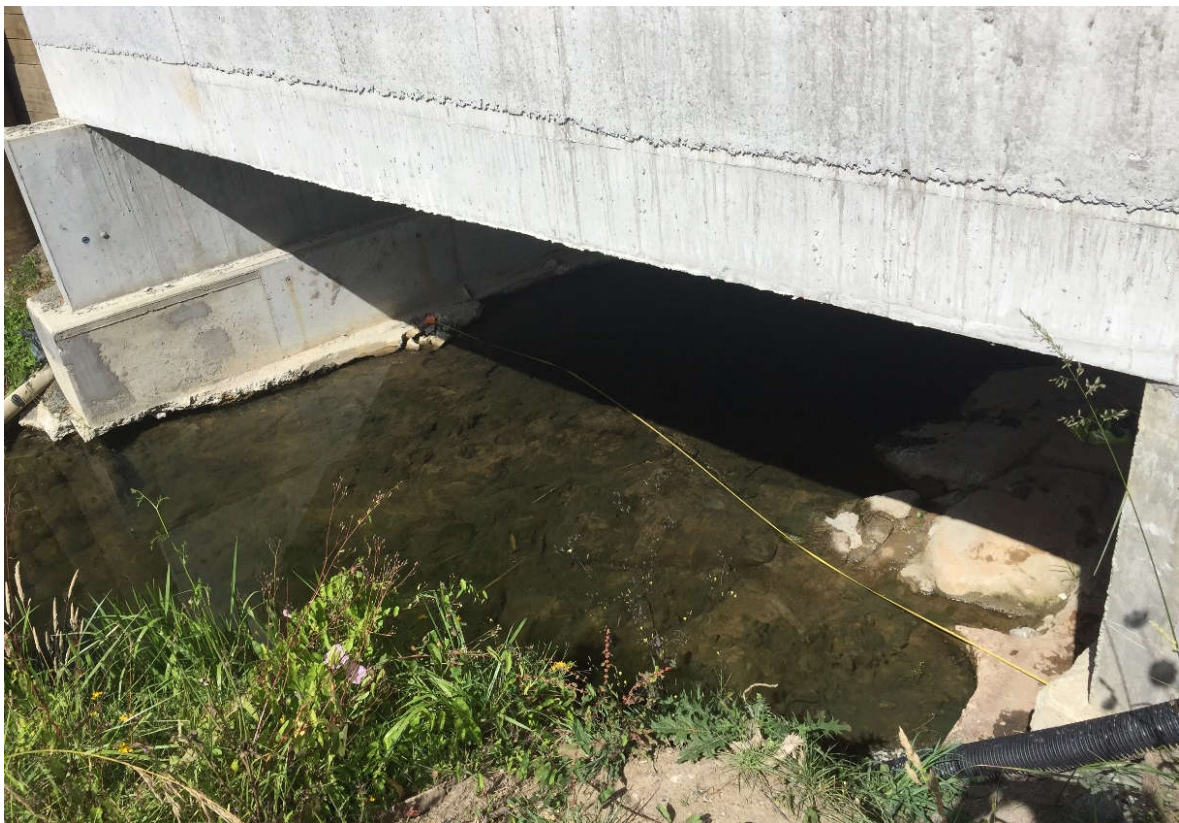
Figure 13 – Falls Road Bridge (Taken by J Curtis 14.01.2017)
