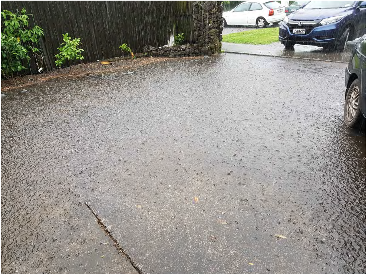
Flooding and cars moved to prevent water damage. The drain grating is under the lemon tree in the centre of the picture and is obviously completely useless in this downpour.
