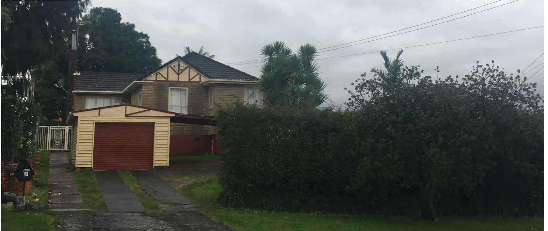
Property 14 Massey Avenue – garage within front yard zone which also has a 2m + hedge
