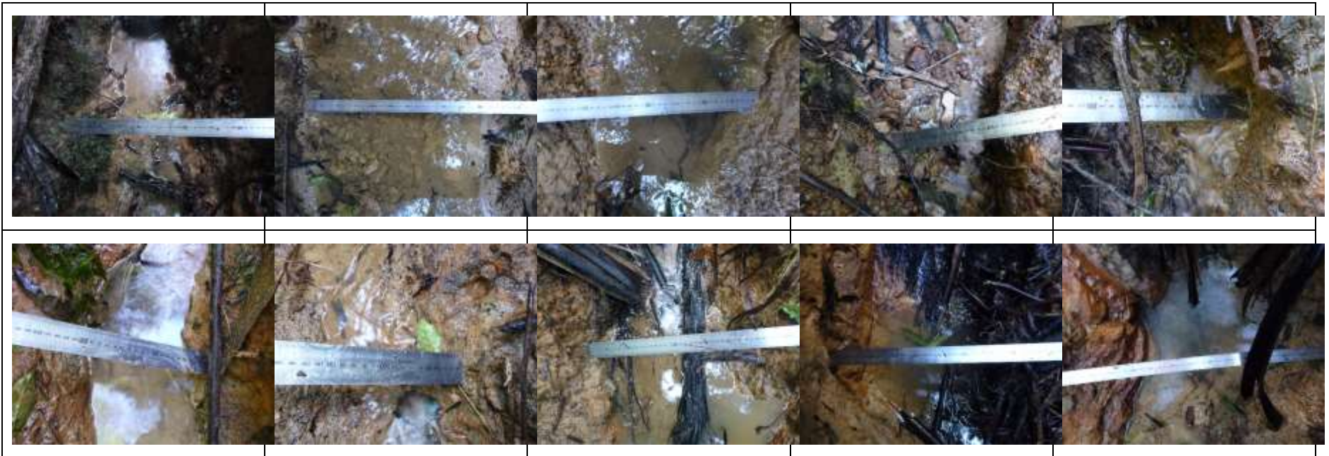
SEV 2 - Southern Block main channel upstream of culvert
