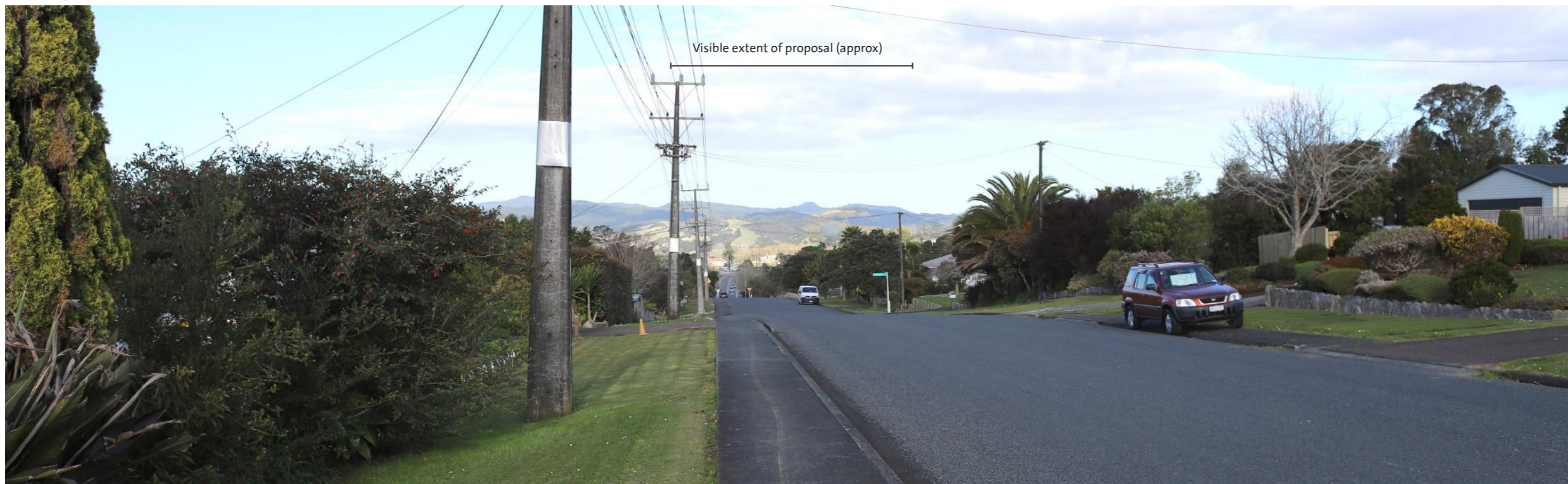
Site Establishment & Initial Construction Works
