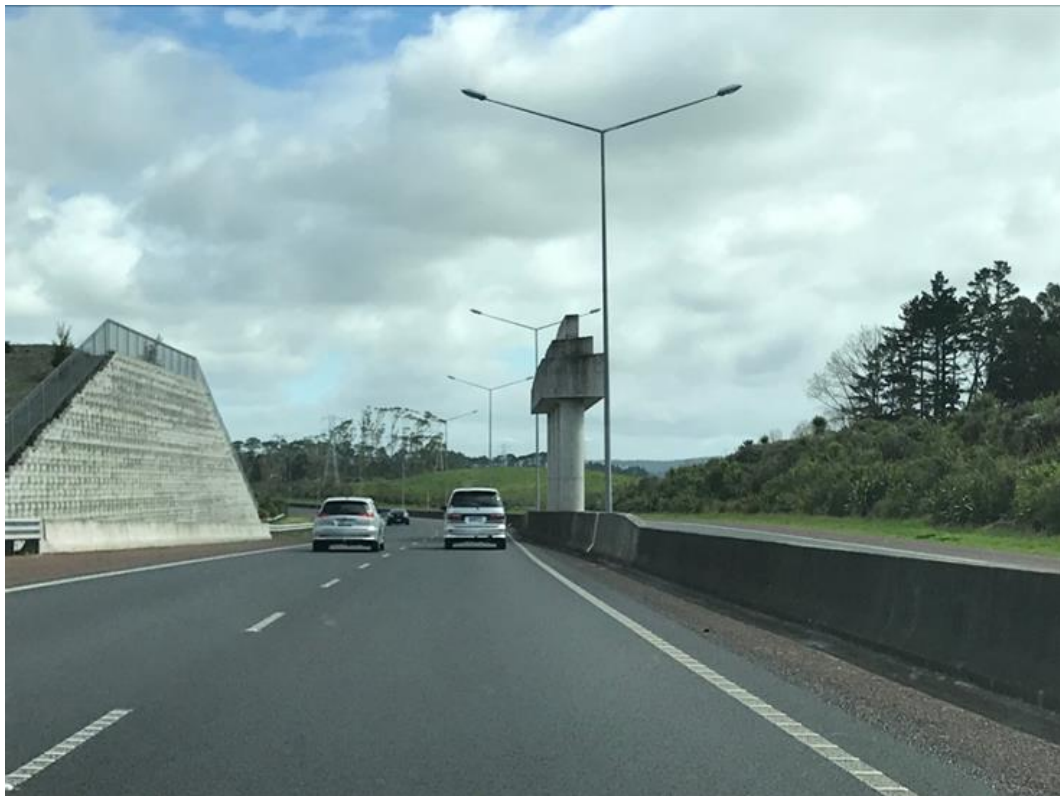
Figure 3: Pillars located on State Highway 16 to support the future Northside Drive extension
