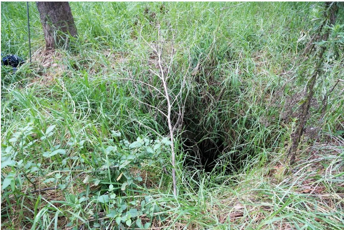
Figure 22. Collapsed entrance point to central emplacement, looking NE
