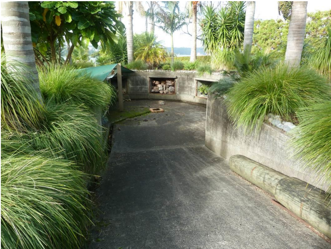
Figure 9. Photograph of the exposed gun emplacement at 19 Scott Road, Hobsonville, looking down the ramp towards the gunpit, with ammunition recesses visible on the far side (photo: Macready 2015)
