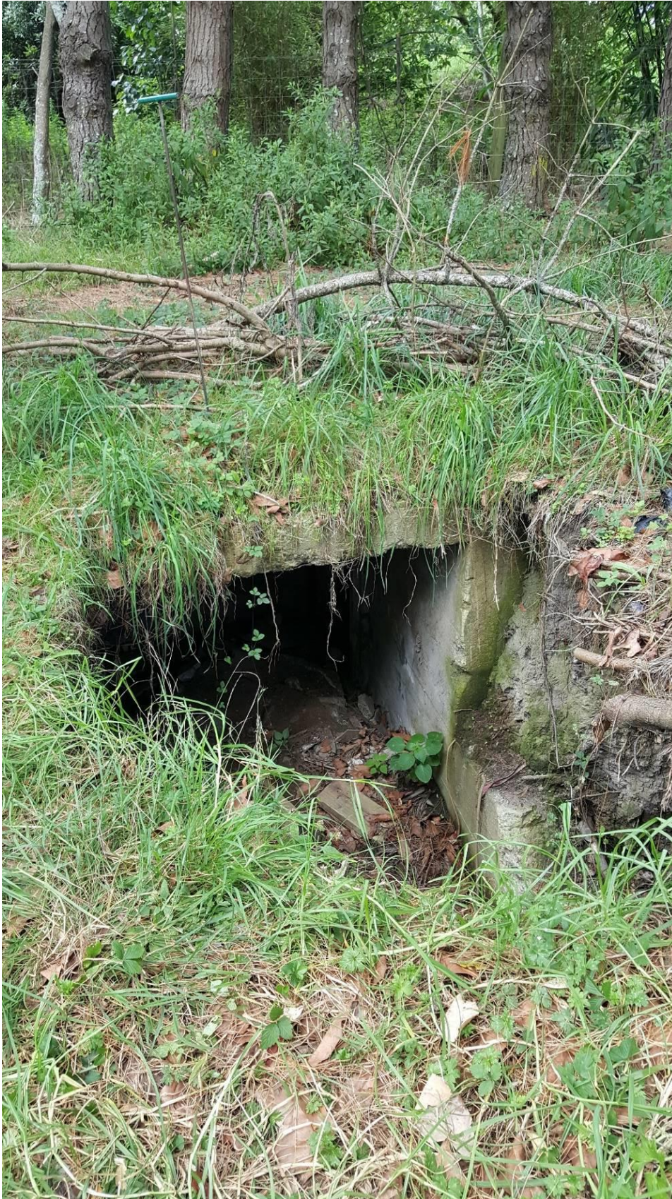
Figure 18. Southern emplacement looking E
