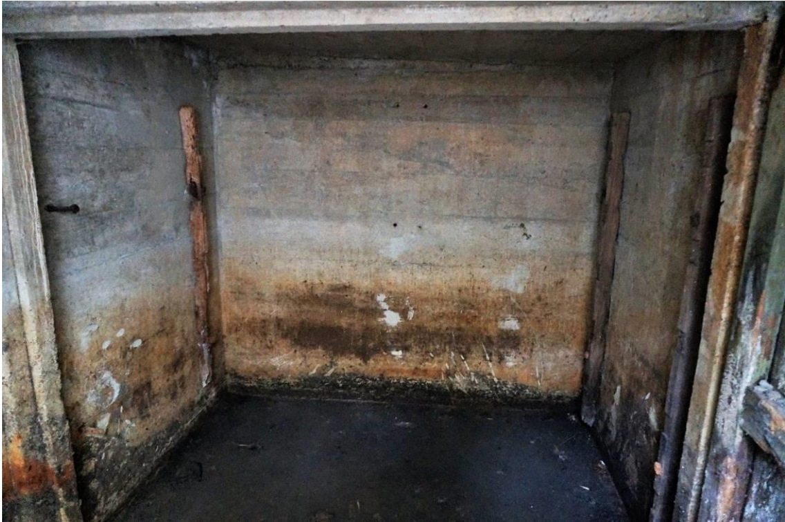
Figure 23. Ammunition recess in central emplacement, looking E/NE
