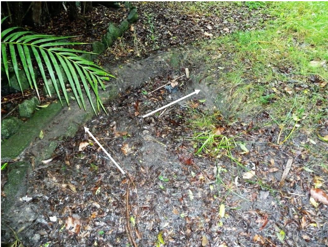
Figure 30. Northern emplacement looking north showing the concrete wall (left arrow) and the one of the locations of subsurface concrete detected through probing (right arrow)
