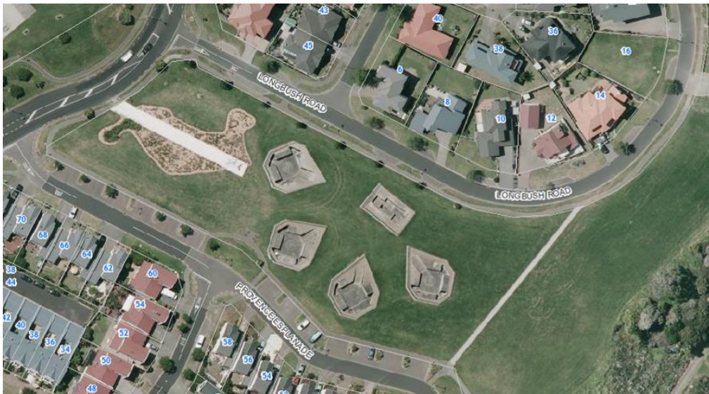
Figure 6. Aerial view of the heavy AA battery at Gunner Drive, Te Atatu (source: Google Maps)
