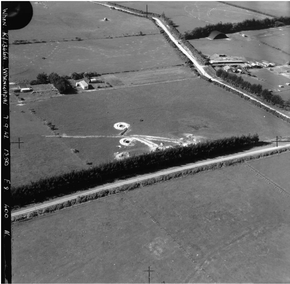
Figure 4. Oblique aerial photo showing the gun emplacements under construction, 7 September 1942 (source: RNZAF Official, K13464)
