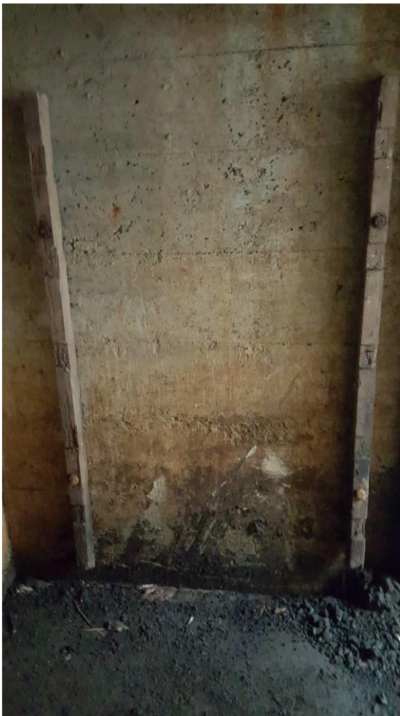
Figure 24. Timber shelving uprights at side of ammunition recess in central emplacement
