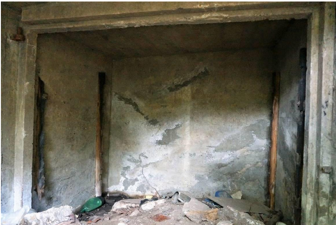
Figure 20. Looking E towards eastern ammunition recess in southern emplacement
