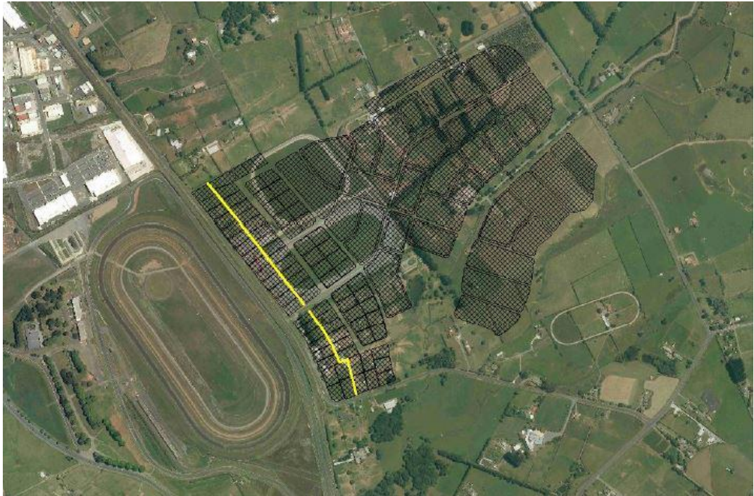
Figure 1: The mid-block' wall
