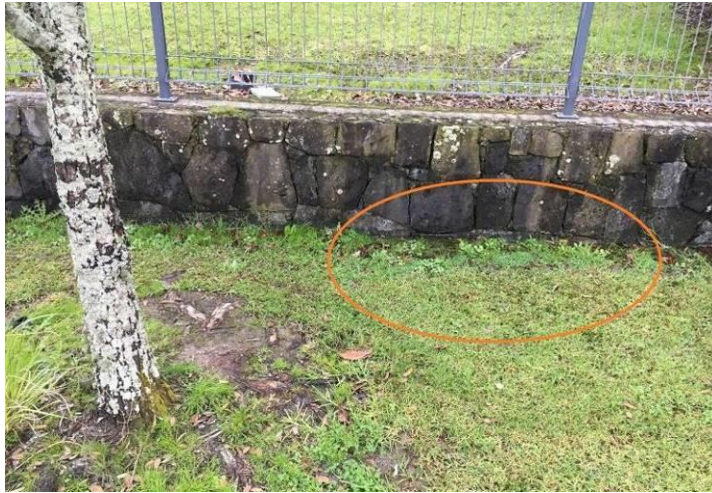
Figure 2 – base of Tree 4, with the location of the historic flowing water that was saturating the roots of Trees 2, 3 & 4 ringed in orange. This water leak was brought to the attention of the tenants within the property, and has since been fixed by a plumber
