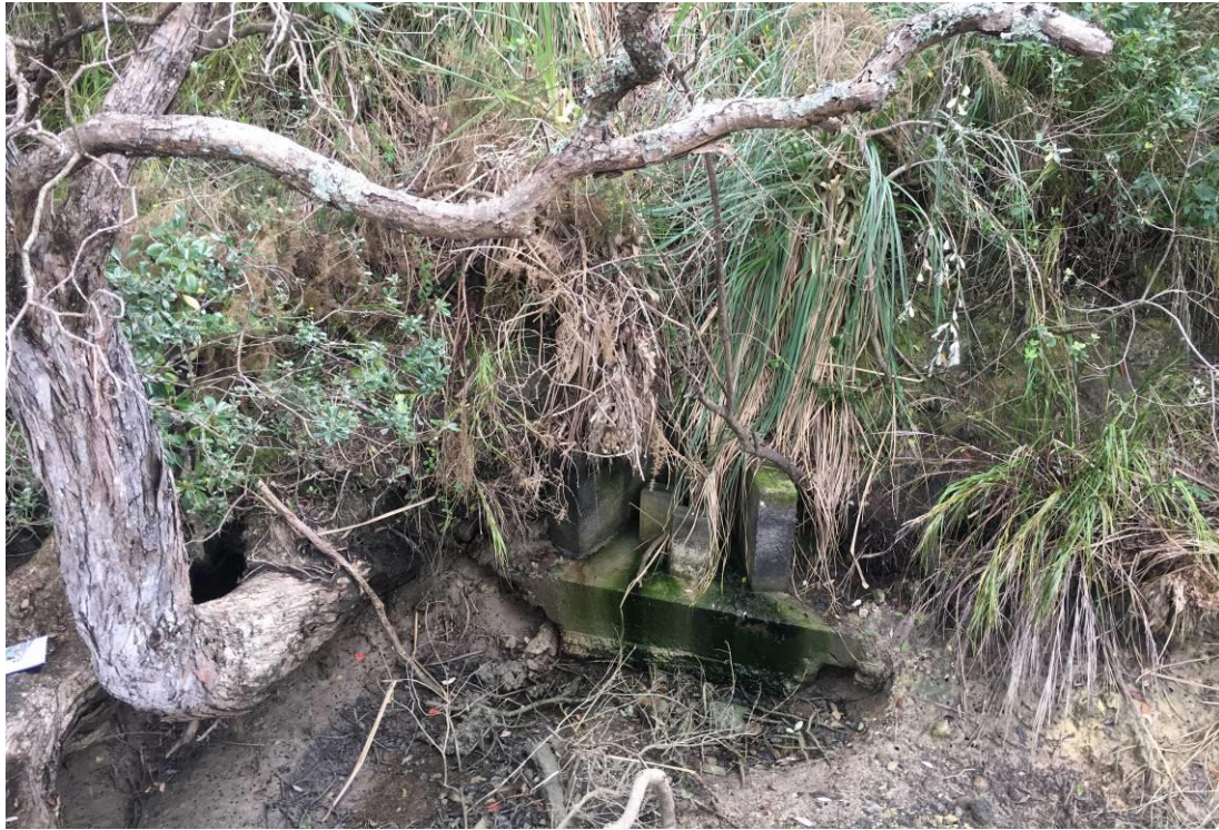
Figure 13 – existing stormwater outlet 2-0
