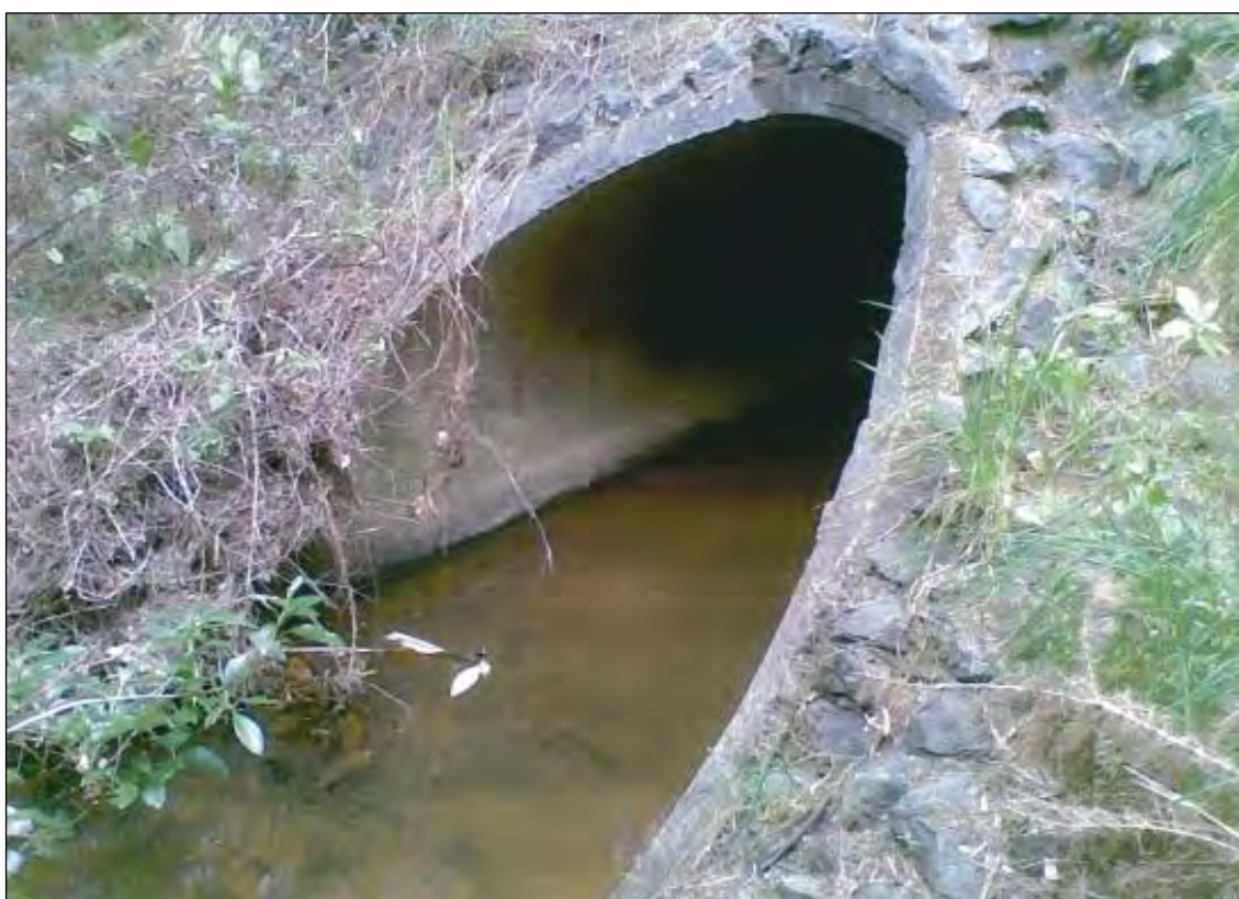
Figure 8: Jack Lachlan Drive culvert.
