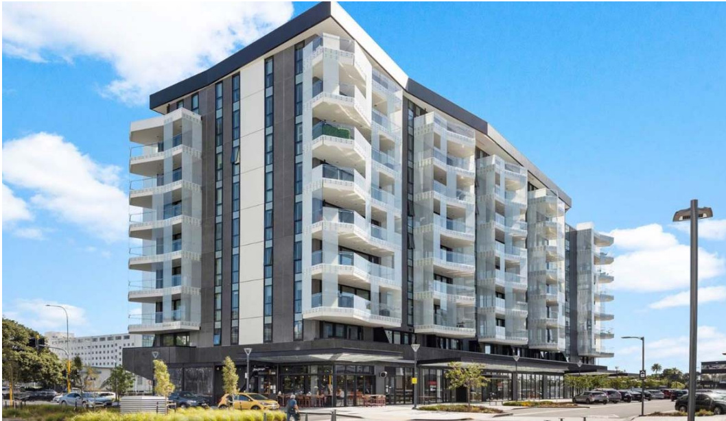
Figure 4: The 9 storey apartment building at 233B Green Lane West.
