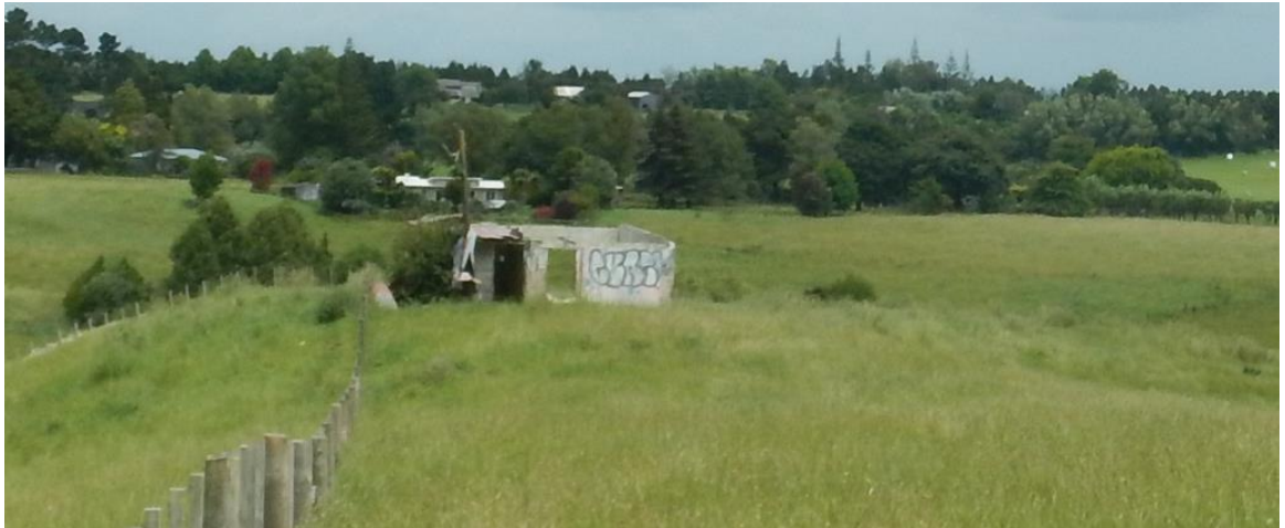
Figure 22. Photograph showing the concrete shed containing the Alfa- Laval Cream Separator in Pt Allotment 15, looking south
