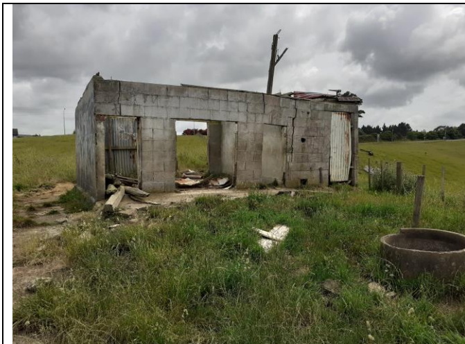
A small concrete shed was identifiable across the central area of the lot. The shed is constructed of concrete cinder blocks.
