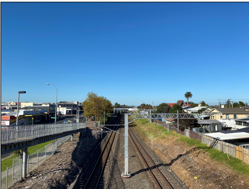
Figure 4-8: NIMT looking south from Papatoetoe Station
