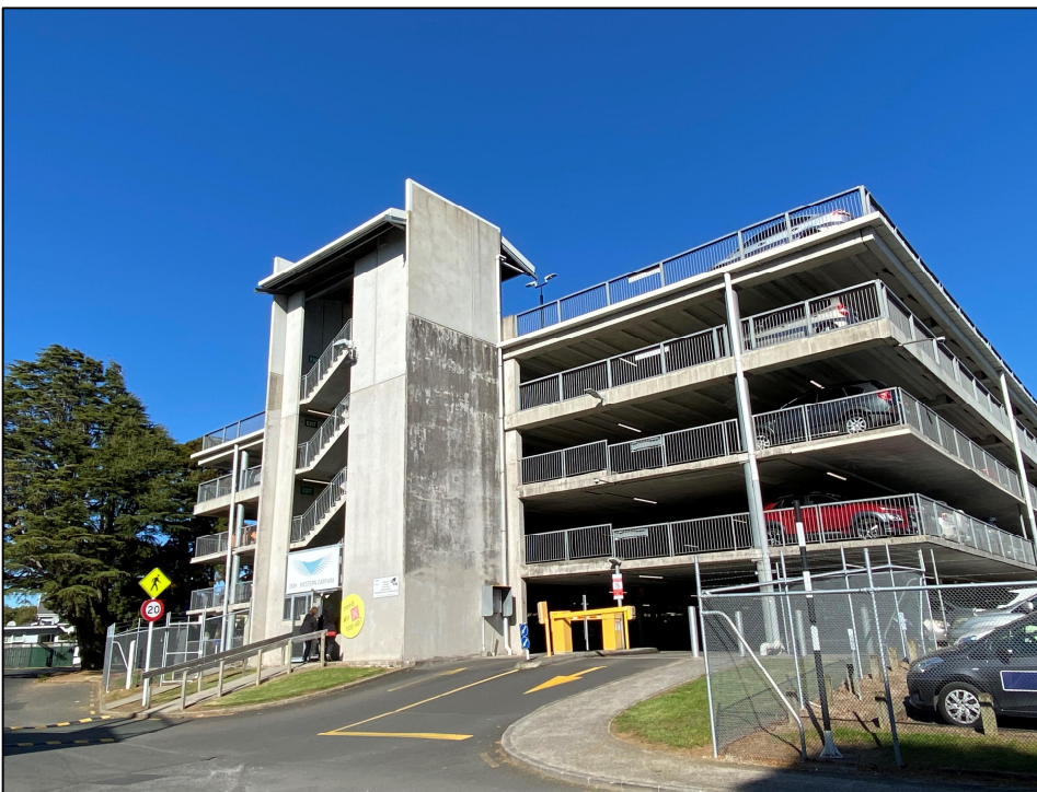
Figure 4-4: Multi-storey car park for hospital staff
