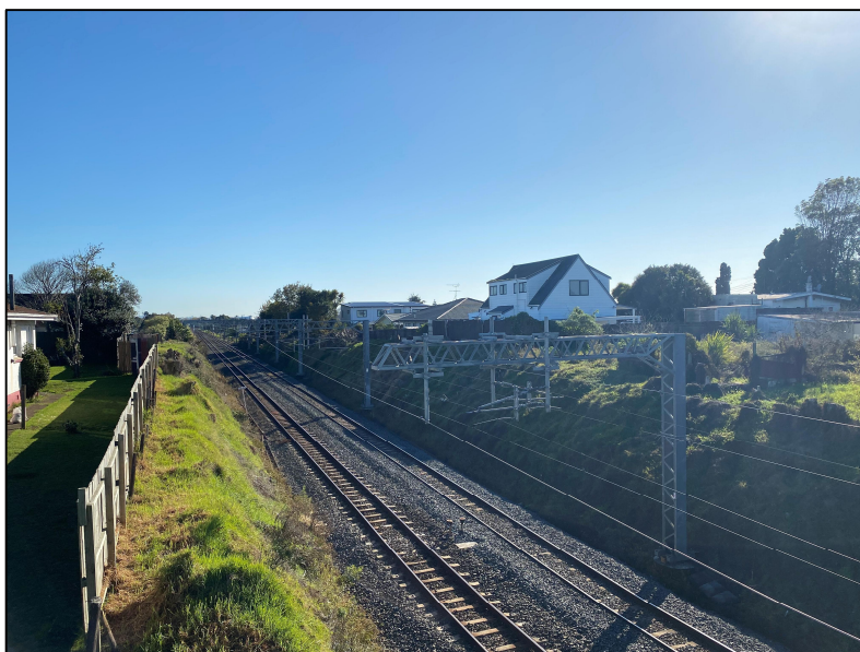
Figure 4-10: View North from Bridge Street
