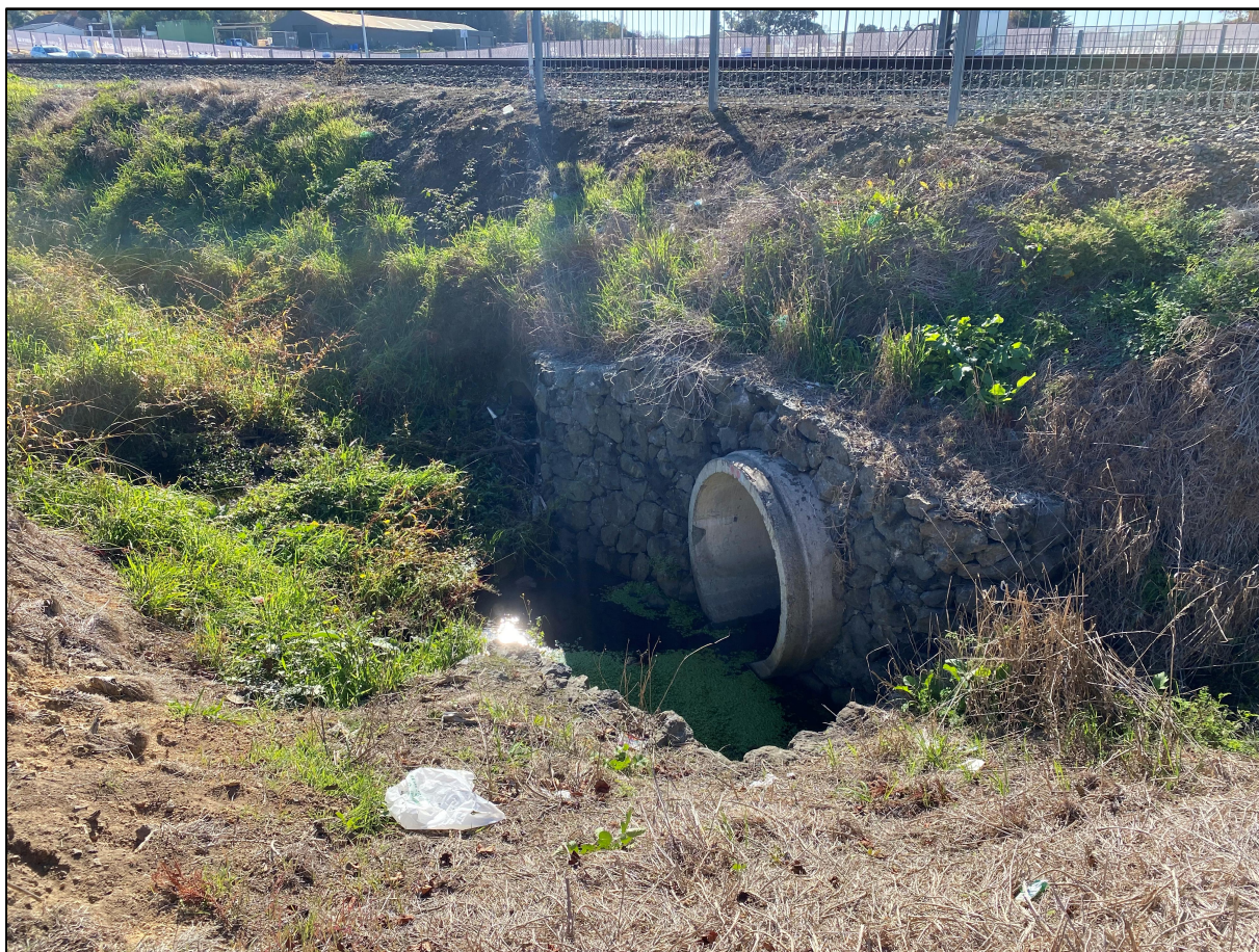
Figure 4-15: Culverts at Middlemore Station
