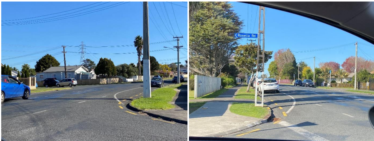
Figure 6-2: View from Rosella Road looking north and south along Orakau Road
