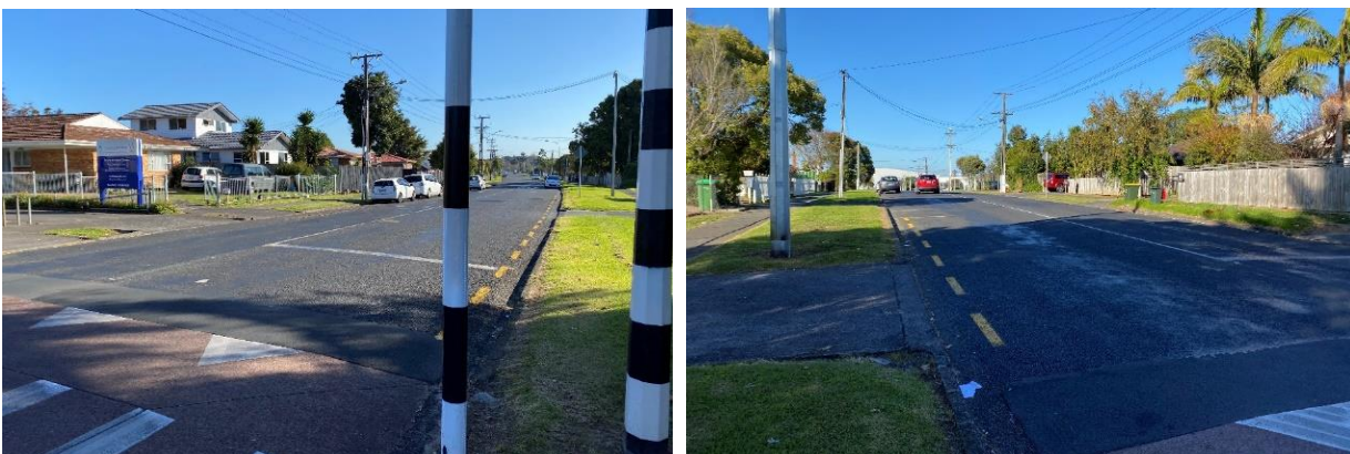
Figure 3-3: Kenderdine Road, looking north from zebra crossing and looking south towards Bridge Street
