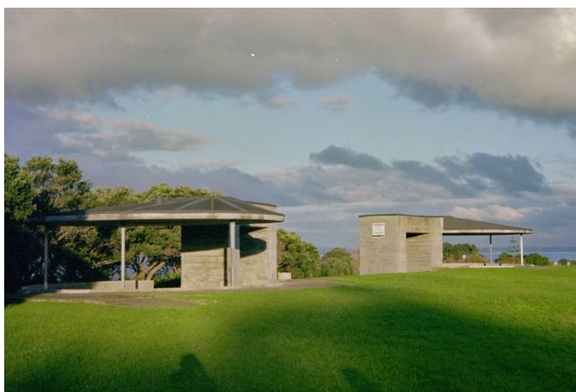
World War II tunnels, Kennedy Park, Castor Bay
