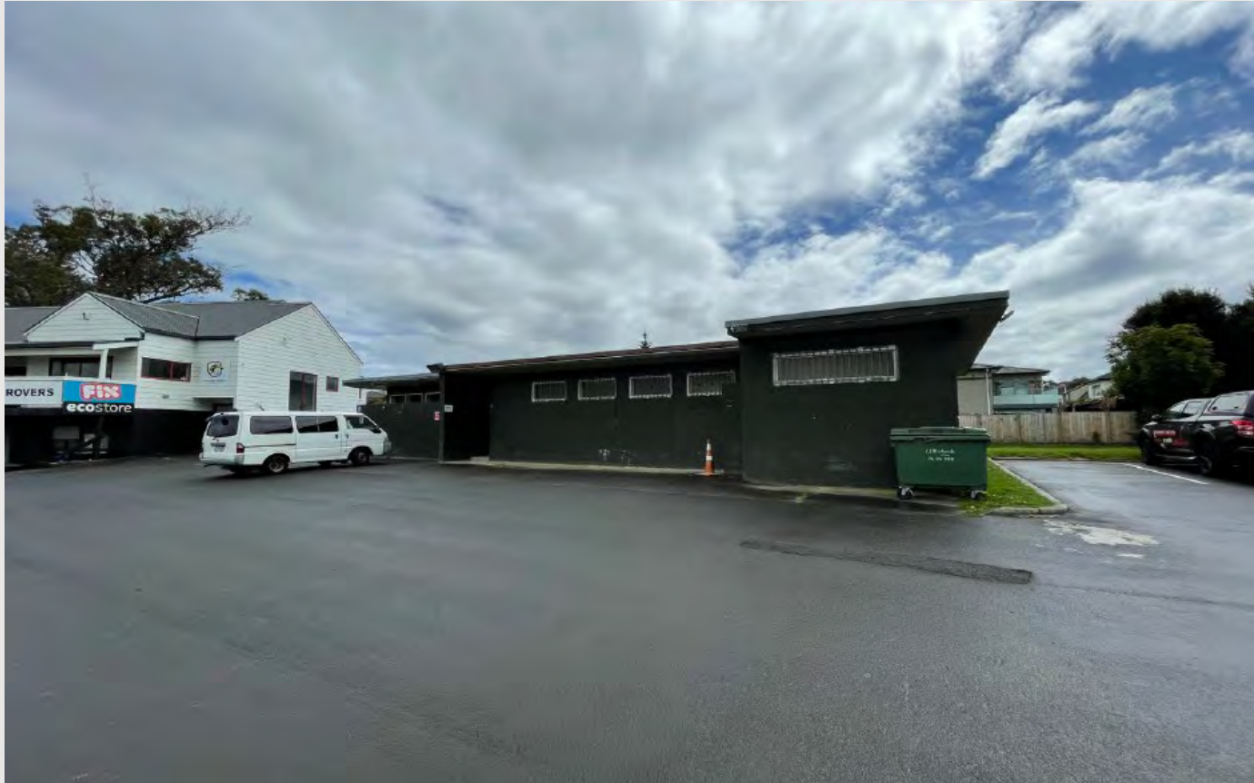
Existing toilets and changing rooms facility
