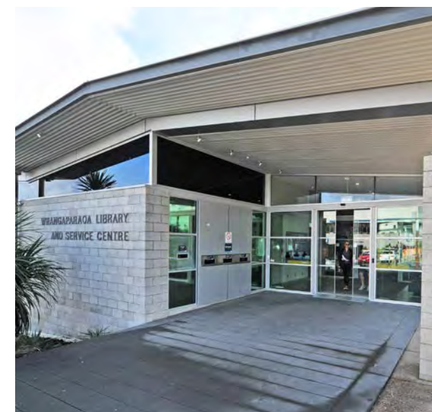
Whangaparāoa Library is an important and well used community building.
