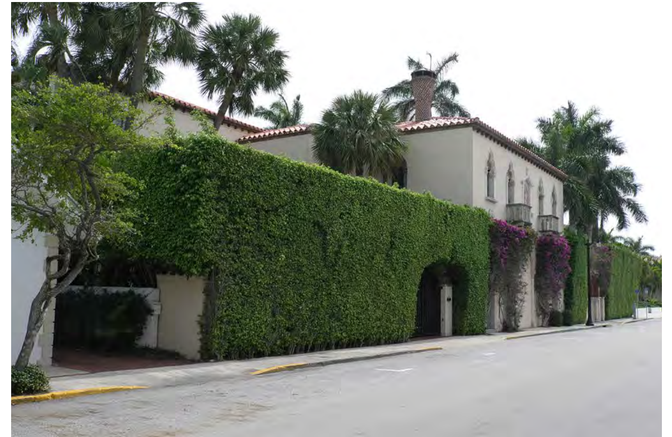
Even anonymous or blank facades can be improved if not 'activated' with appropriate landscape treatments.
