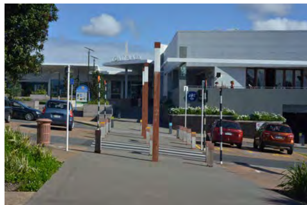
Present connection between library and Coast Plaza – functional but not high quality.
