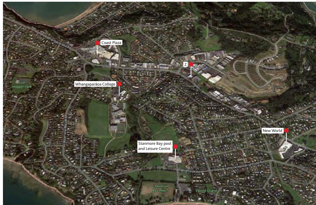
Coast Plaza identifies the town centre hill side location. New World supermarket right of picture is the location of the most recent larger scale commercial development close to the town centre.
