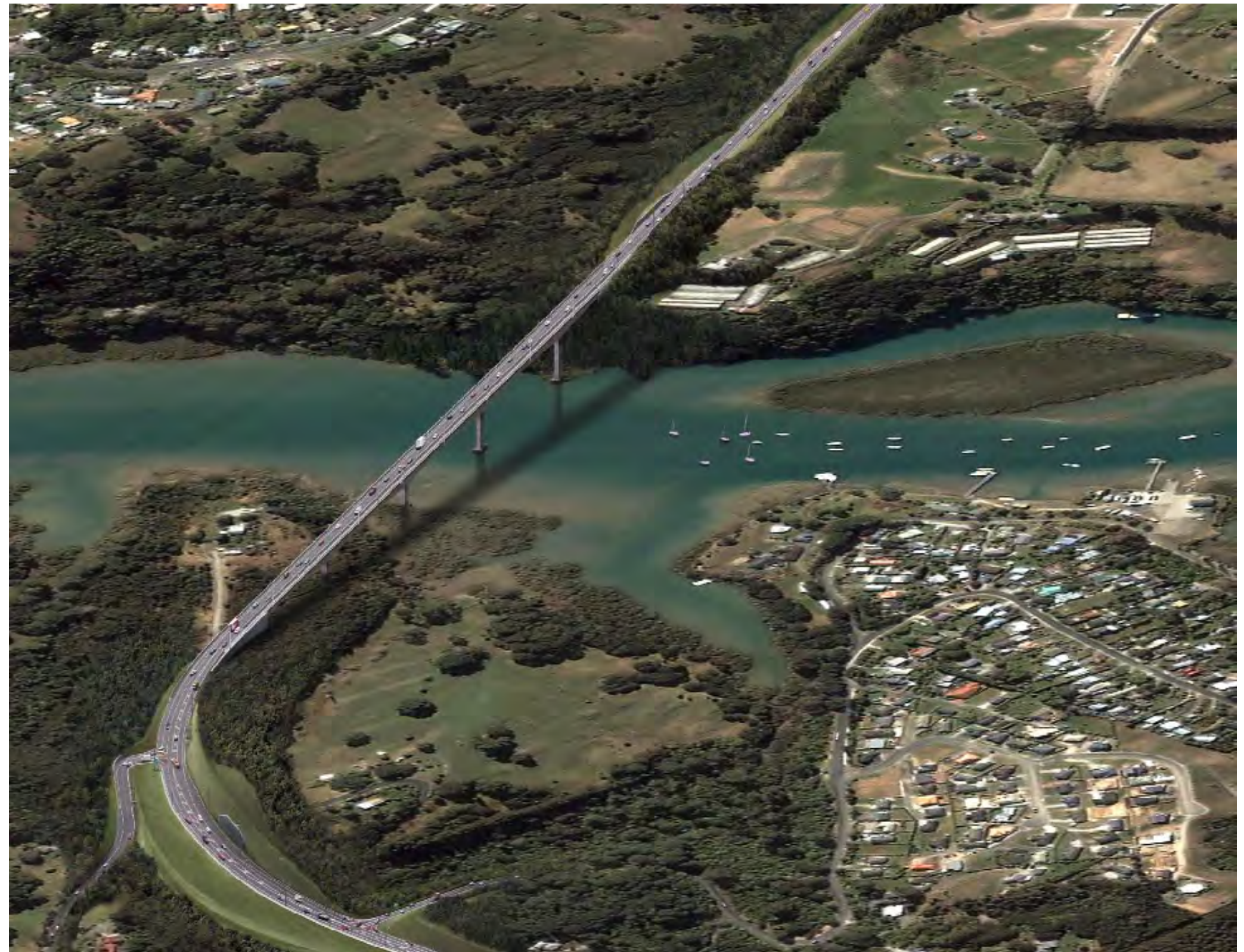
The bridge that is planned as part of Penlink.
