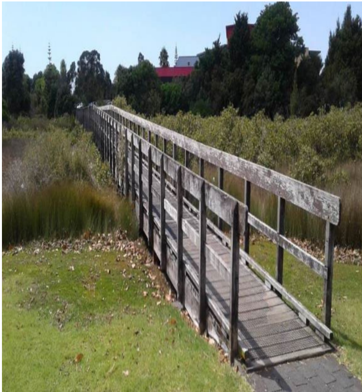
Original bridge prior to the renewal
