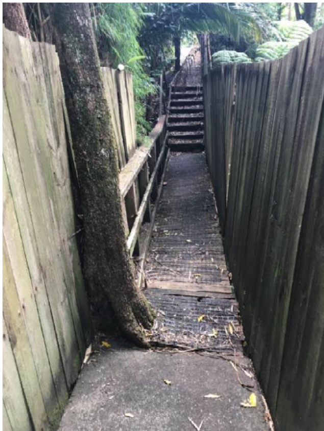
Original bridge prior to the renewal
