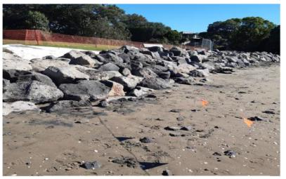
Placing rocks over geotextile membrane
