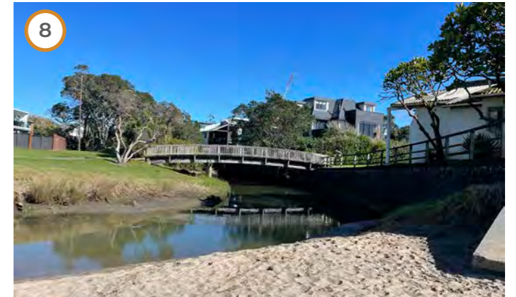
Looking west towards the bridge connecting the north and south sections of the Mairangi Bay Beach Reserves
