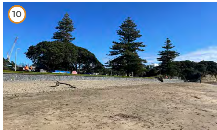
Looking west towards the Mairangi Bay Beach Seawall
