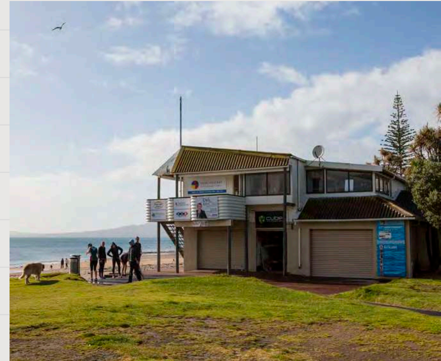
Above image - MBSLC building. Source: Auckland Council's The Wire intranet site.
