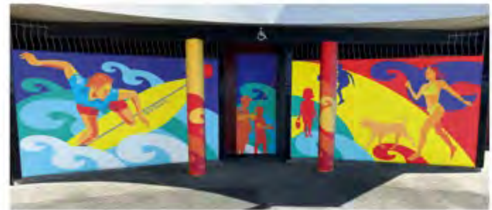
Toilet walls, door and posts
