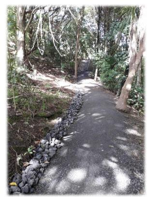
Aggregate surface with rock channel
