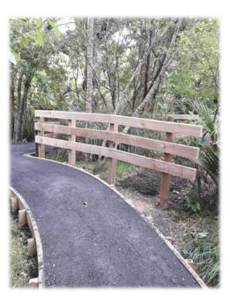
Aggregate surface with Edge Board
