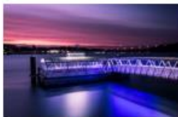
Beach Haven Ferry Terminal.
