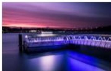
Beach Haven Ferry Terminal.
