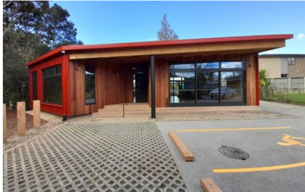
Kaipātiki Project at Lauderdale Rd, Birkdale - renew/re build facility
