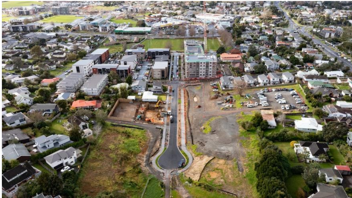
Kaka St progress. Road widening works completed by Piritahi in June.
