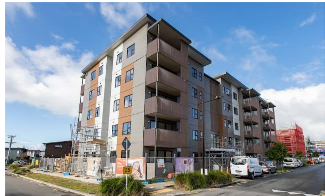
View from Tonar St, 5 level walk-up apartment completed shortly
