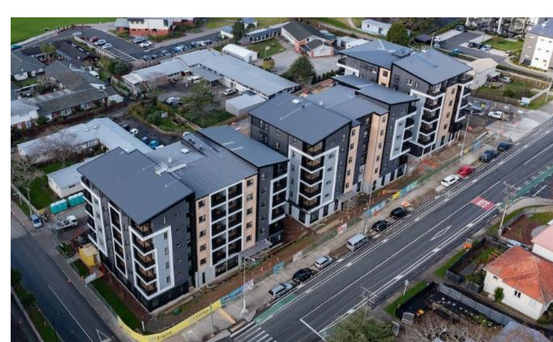
Lake Rd Kāinga Ora apartments in construction
