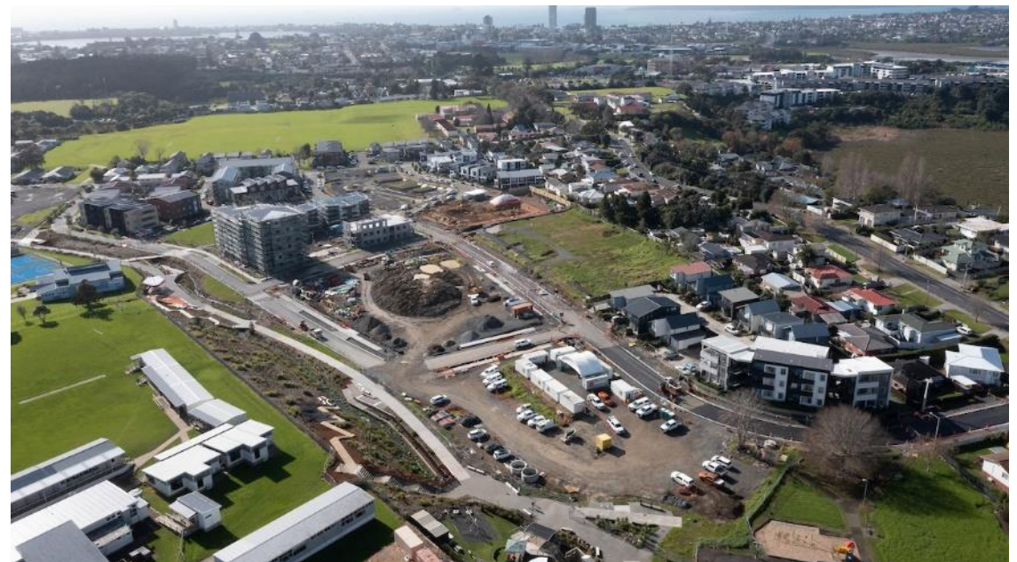
Piritahi Stage 5 Cadness St work progress.
