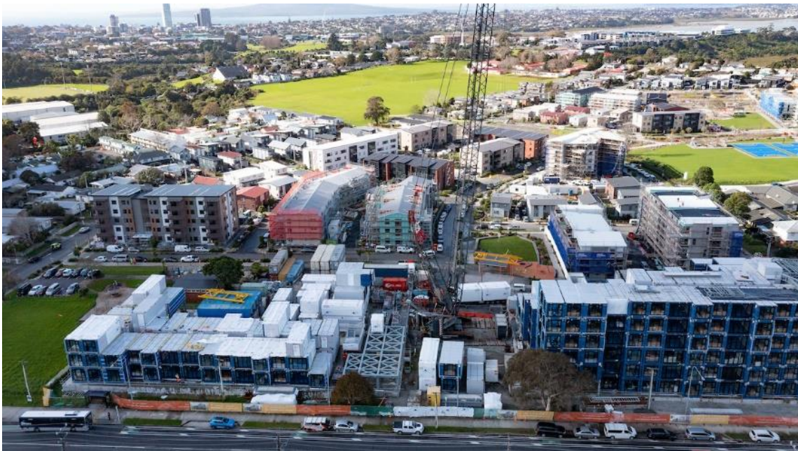
TLC Lake Road apartment construction progress.
