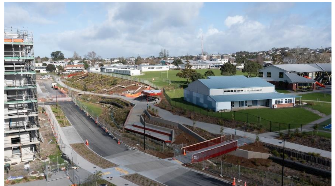
Te Ara Awataha School's edge and surrounding Piritahi work progress.
