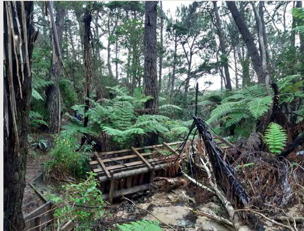
Missing bridge relocated 15m down stream
