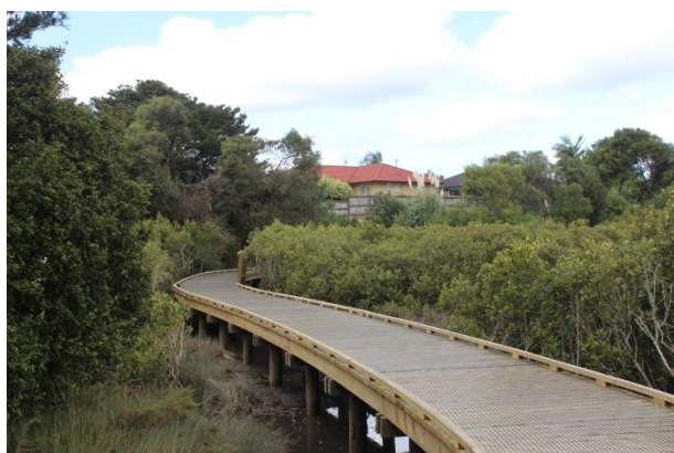
Figure 22: Waimahia Inlet boardwalk
