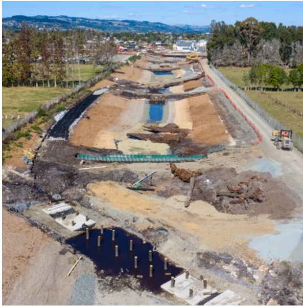
Awakeri Wetlands under construction
