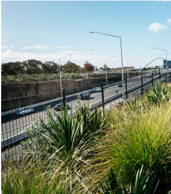
Cycleway alongside SH20.
