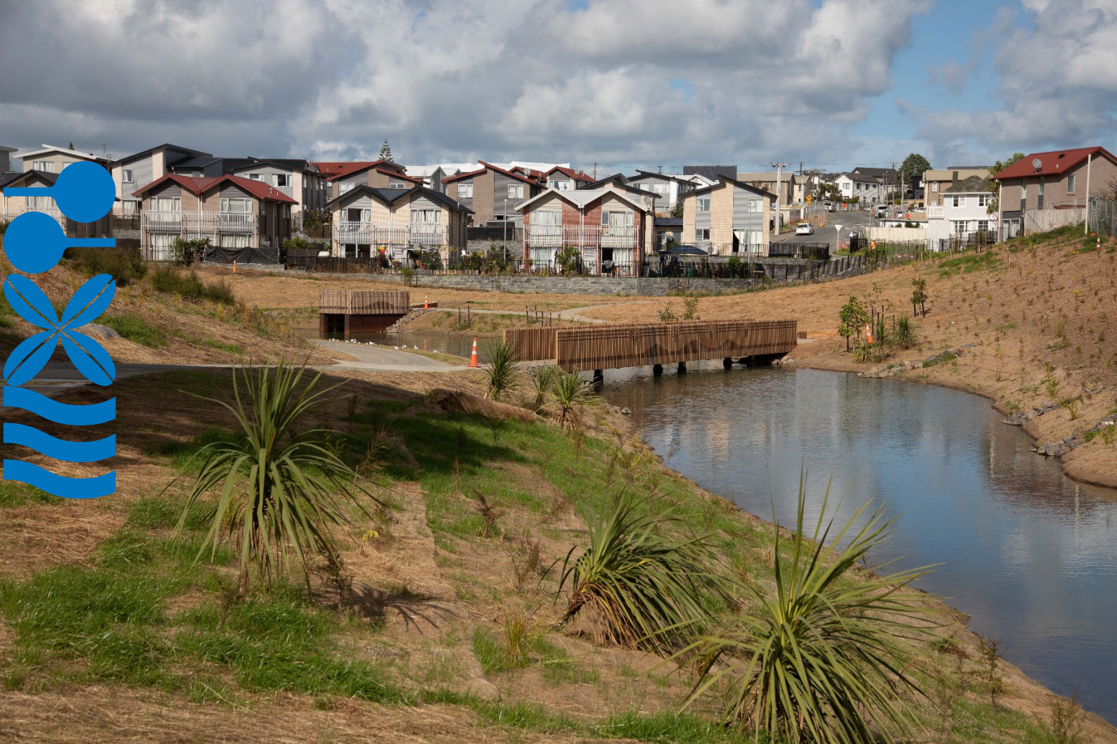
Freeland Reserve upgrades freshly completed
