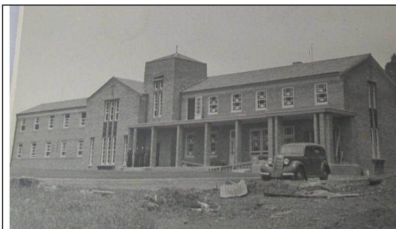
Additions to the western end of the Friary nearing completion. Source: Auckland Council Archives MRB 11D, H15, Pt 6, Box 16.
