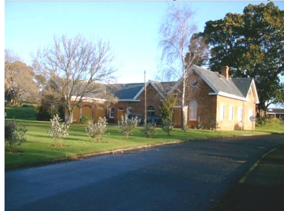
Stables at The Pah, 72 Hillsborough Road, Hillsborough
