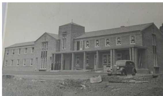
Figure 43: Additions to the western end of the Friary nearing completion. Source: Auckland Council Archives MRB 11D, H15, Pt 6, Box 16.
