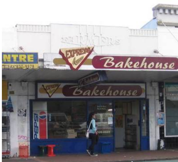
Figure 20: 985 Dominion Road. The original drawings dated November 1940, for the Farmers Building show that the building was for R H Page contractor, and were prepared by R H Page.
