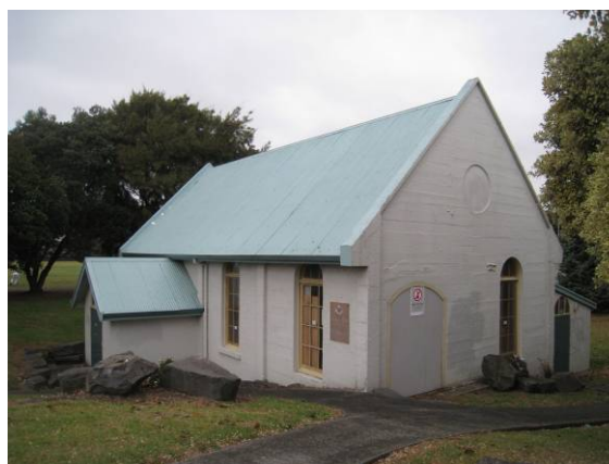
Figure 50: Three Kings Pumphouse. Matthews & Matthews Architects Ltd, 2010.
