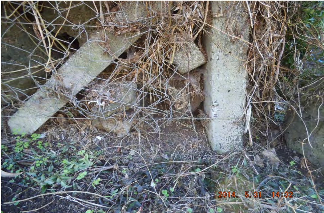
Figure 60 Concrete reinforced posts with stay and wire and netting imbedded into section of wall dissected by Right of Way. Image taken by John Adam in June 2014 Photograph no. DSCF 0366
