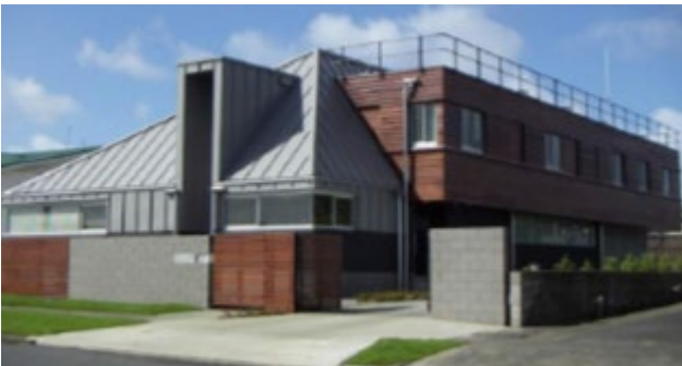
Elcoat Emergency Coordination Centre (ECC)
