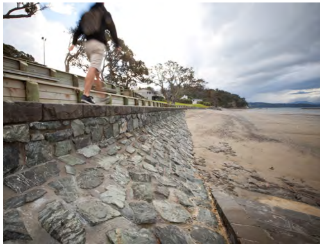
Coastal Seawall Algies Bay
