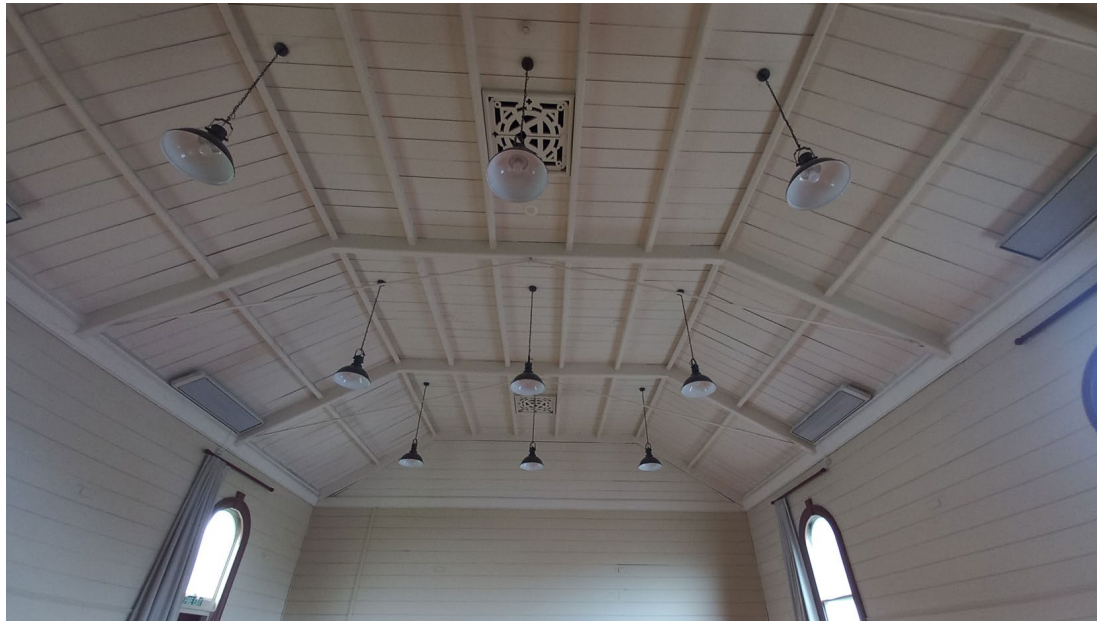
New lighting fixtures and configuration in the main hall
