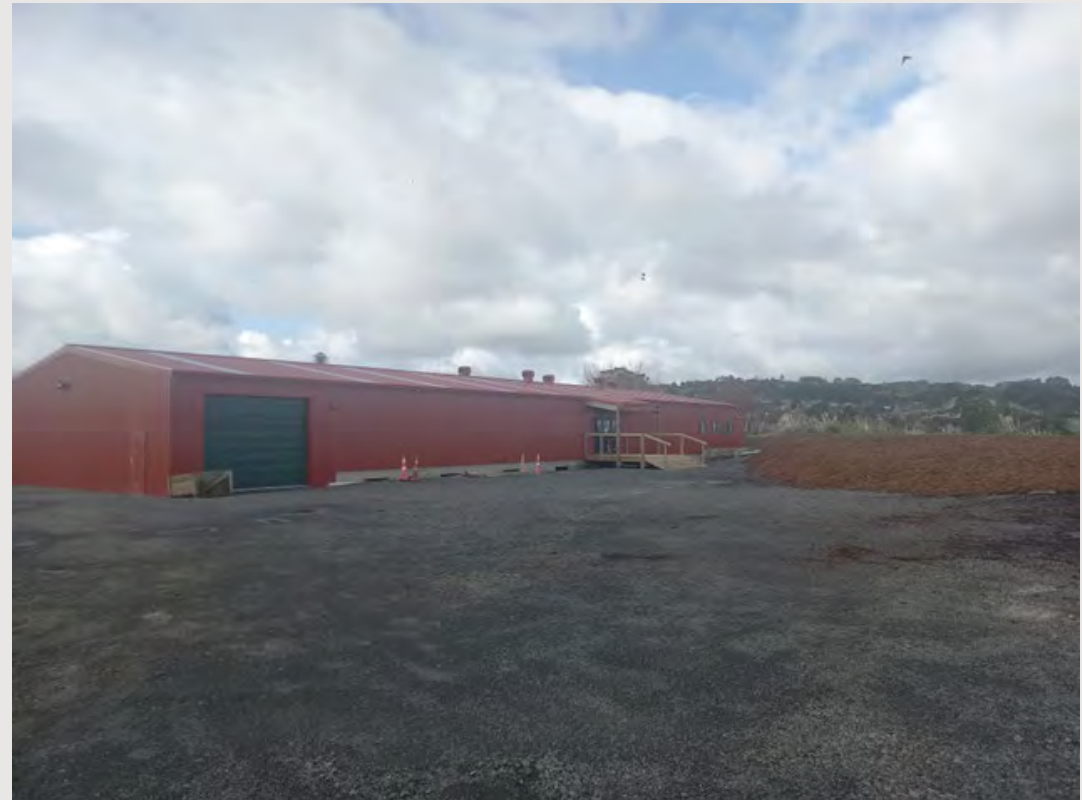
Rear of shop and carpark area
